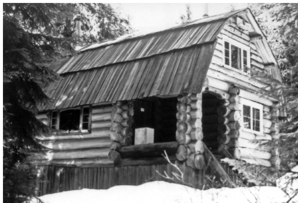
Fig 3 Challenger Inn (235) Log structure, shake barn roof
