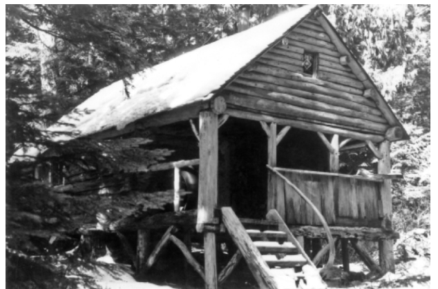
Fig 4 Pastime (240) Log structure, cedar shake peak roof
