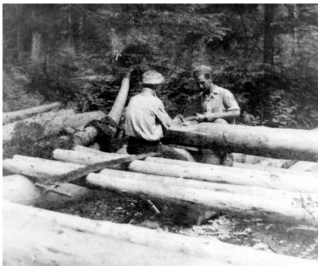
Fig 7 Making a joint. These are floor strings that the saw is on (A. Charboneau collection 1936)
