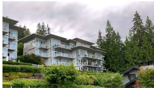
Boulders, West Vancouver
