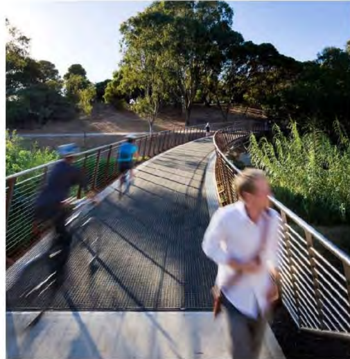
River Torrens Bridge, Australia
