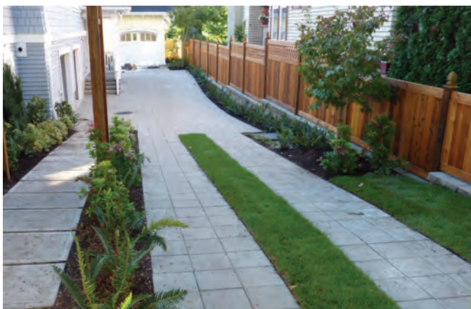
Fig 2.8: Where driveways are required, consider alternative paving materials that reduce runoff.
