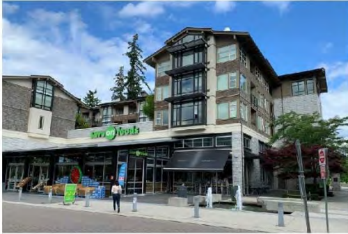
Wesbrook Village, Vancouver
