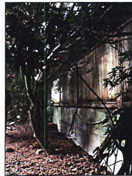
TYPICAL RETAINING WALL CONDITION ALONG SIDE YARDS
