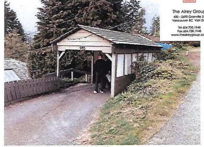
VIEW OF EXISTING CARPORT FROM LANE
