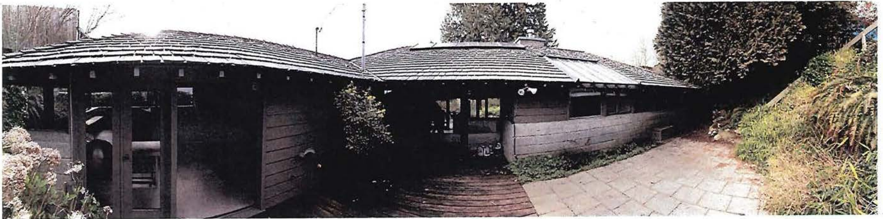
PANORAMIC VIEW OF NORTH ELEVATION
