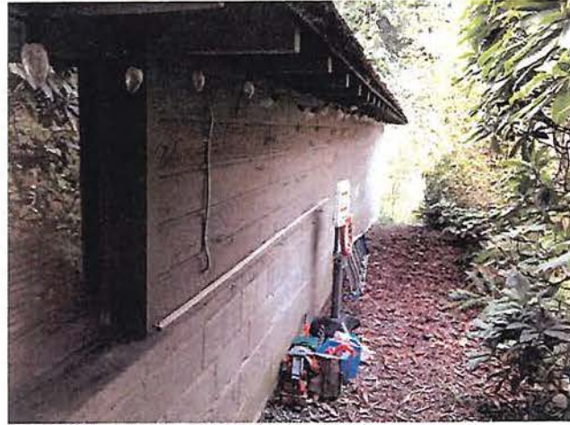
VIEW LOOKING NORTH ALONG EAST ELEVATION
