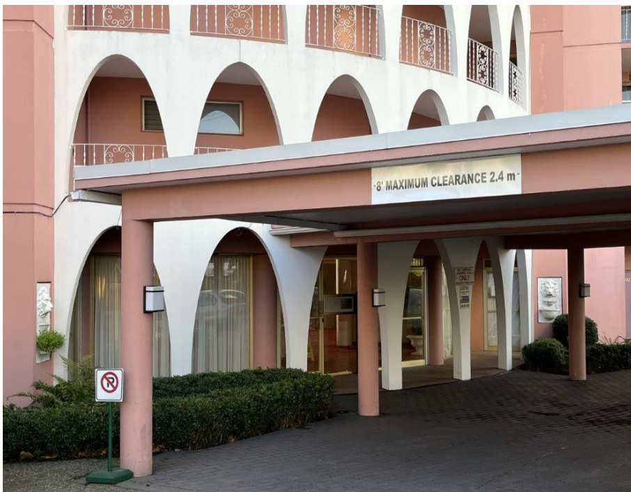
Figure 3 Porte cochere and entry, 2024. Photo by Jennifer Clay
