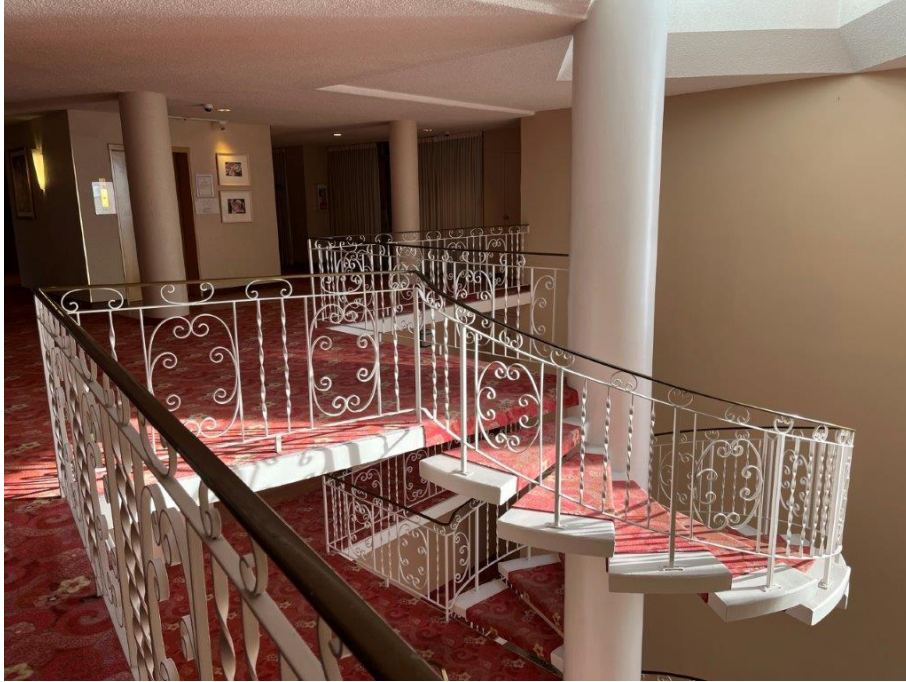
Figure 7 Interior floating stair with decorative railing, 2024. Photo by Jennifer Clay
