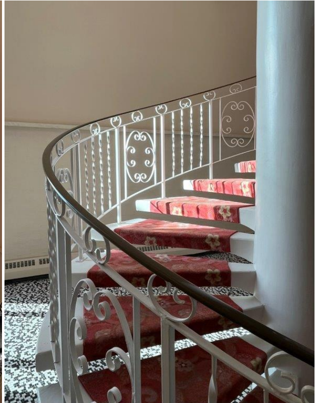
Figure 9 Floating stair, 2024. Photo by Jennifer Clay
