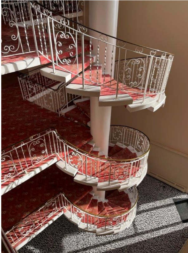
Figure 8 Floating stair, 2024. Photo by Jennifer Clay
