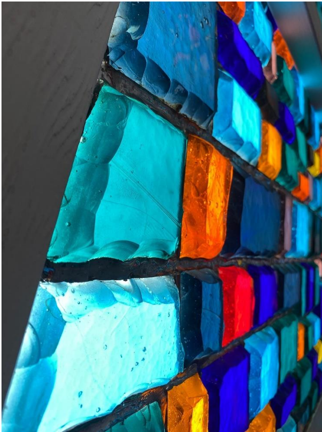
Close-up of the faceted dalle slab glass by Bold interior 'walls of colour' faceted slab-glass windows by the Rault Freres of Renne, France Photo: West Coast Modern League
