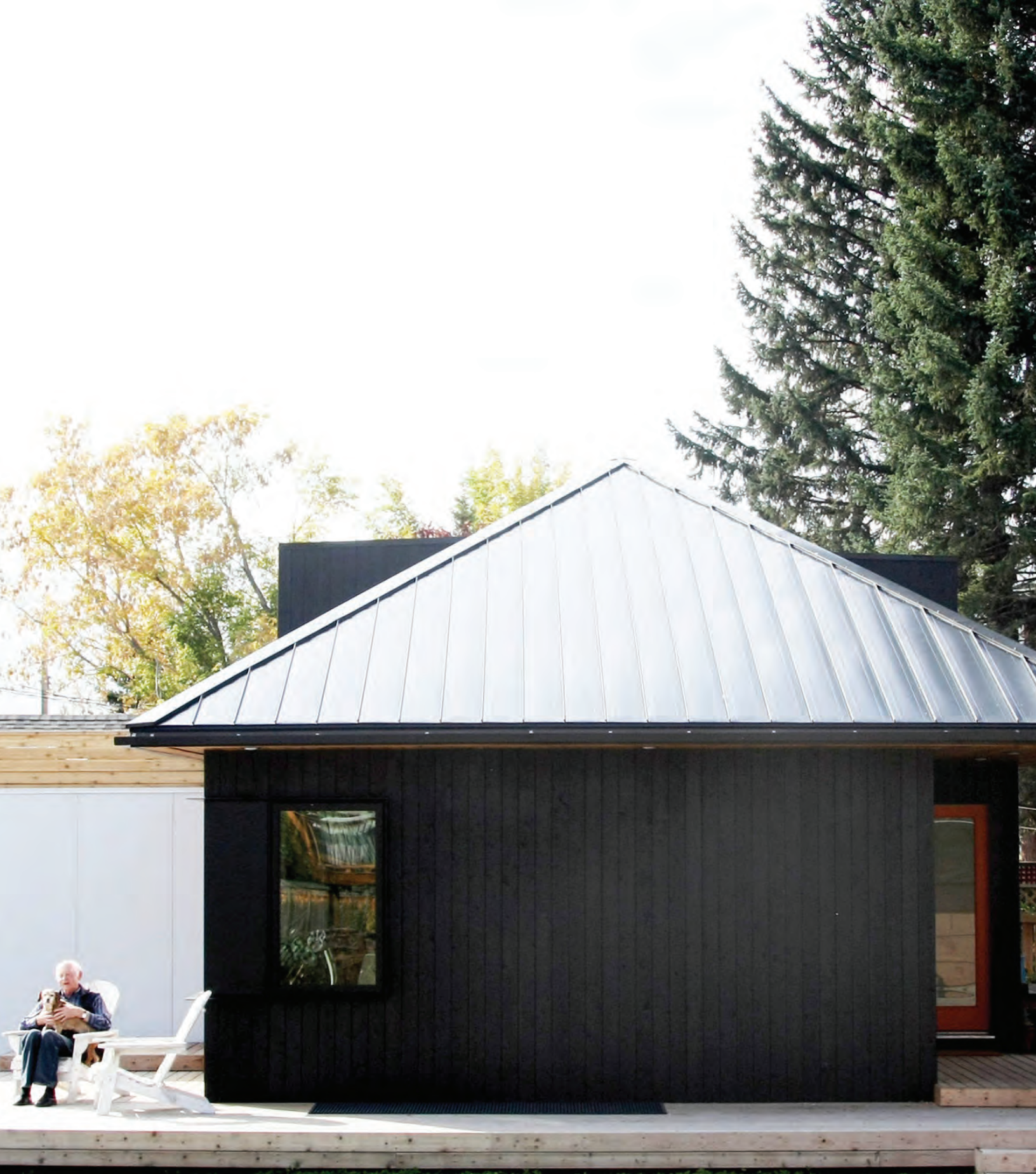
Fig 3.0: Single-storey coach house with high quality materials and functional outdoor space allows for aging in place.
