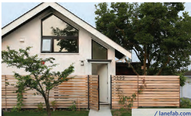
Fig 1.1: Example of a well detailed, modest coach house that illustrates residential character and identity.
