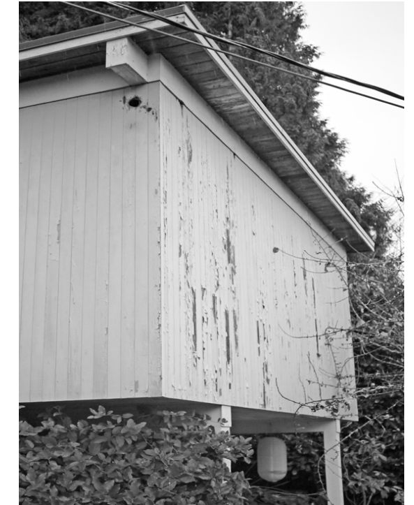
View of Existing Garage from Garden
