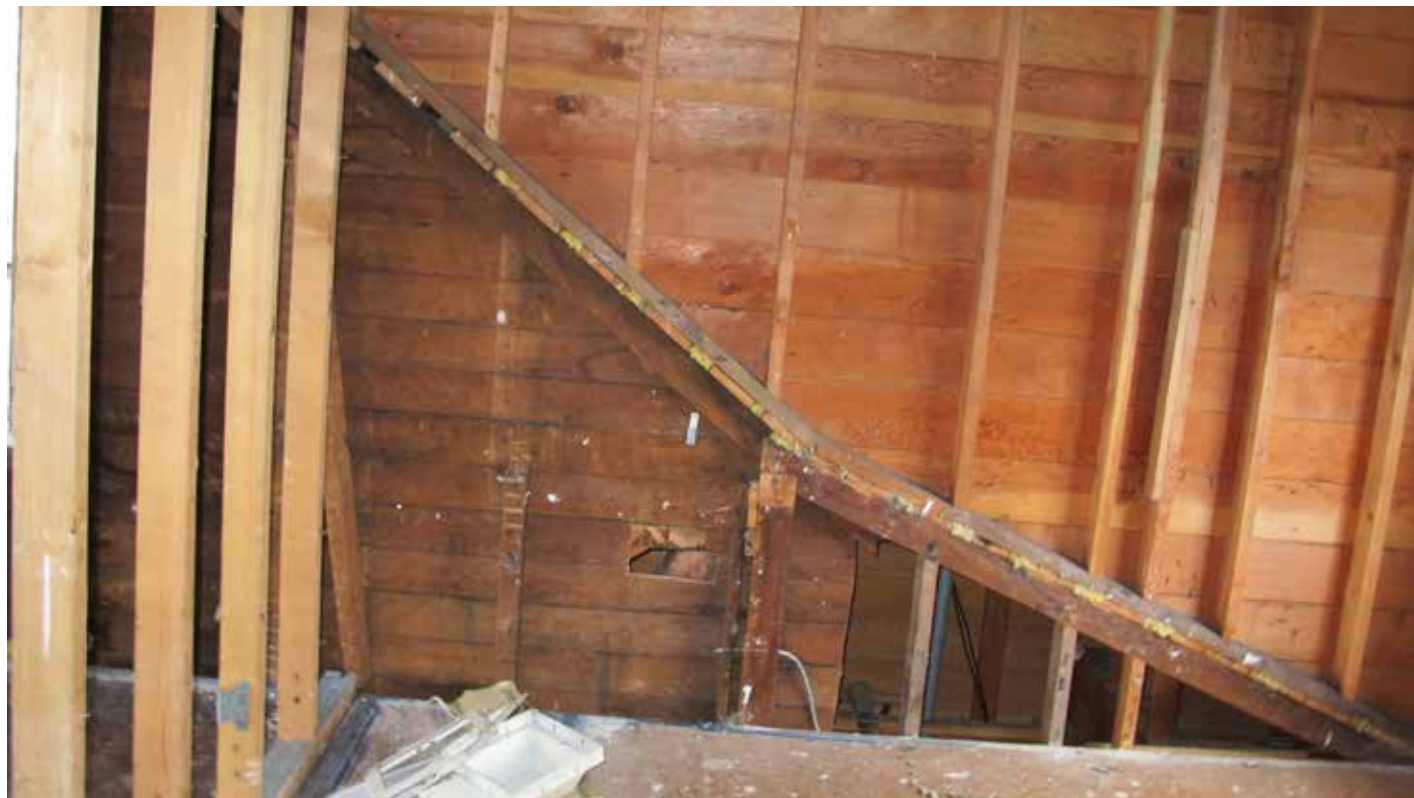
Siding behind later construction, Ground Floor East Side
