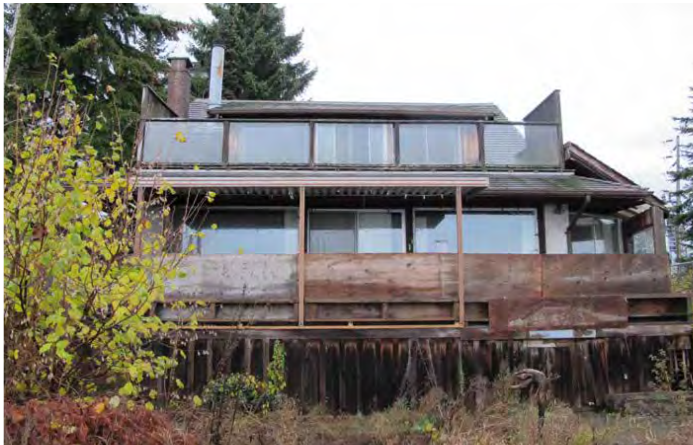
Existing South Elevation. November 2020
