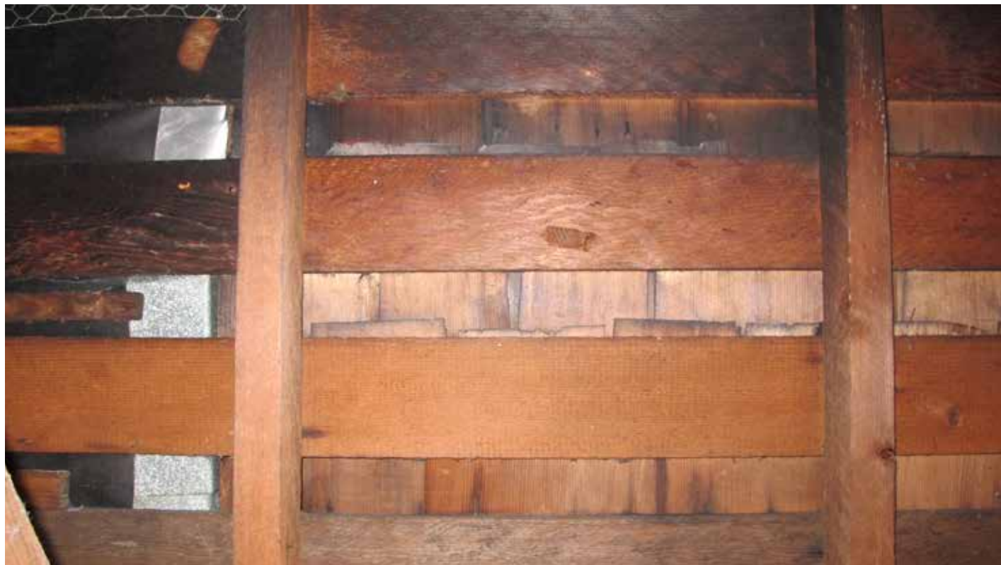
Underside of intact cedar shingle roofing
