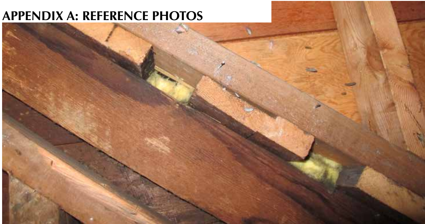
Cut-through roof structure showing original nailing strips.
