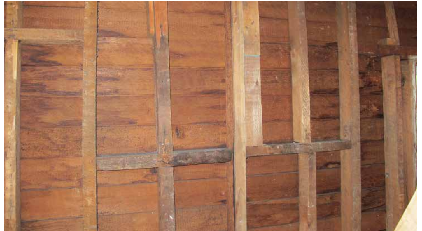
Backside of exterior cladding.
