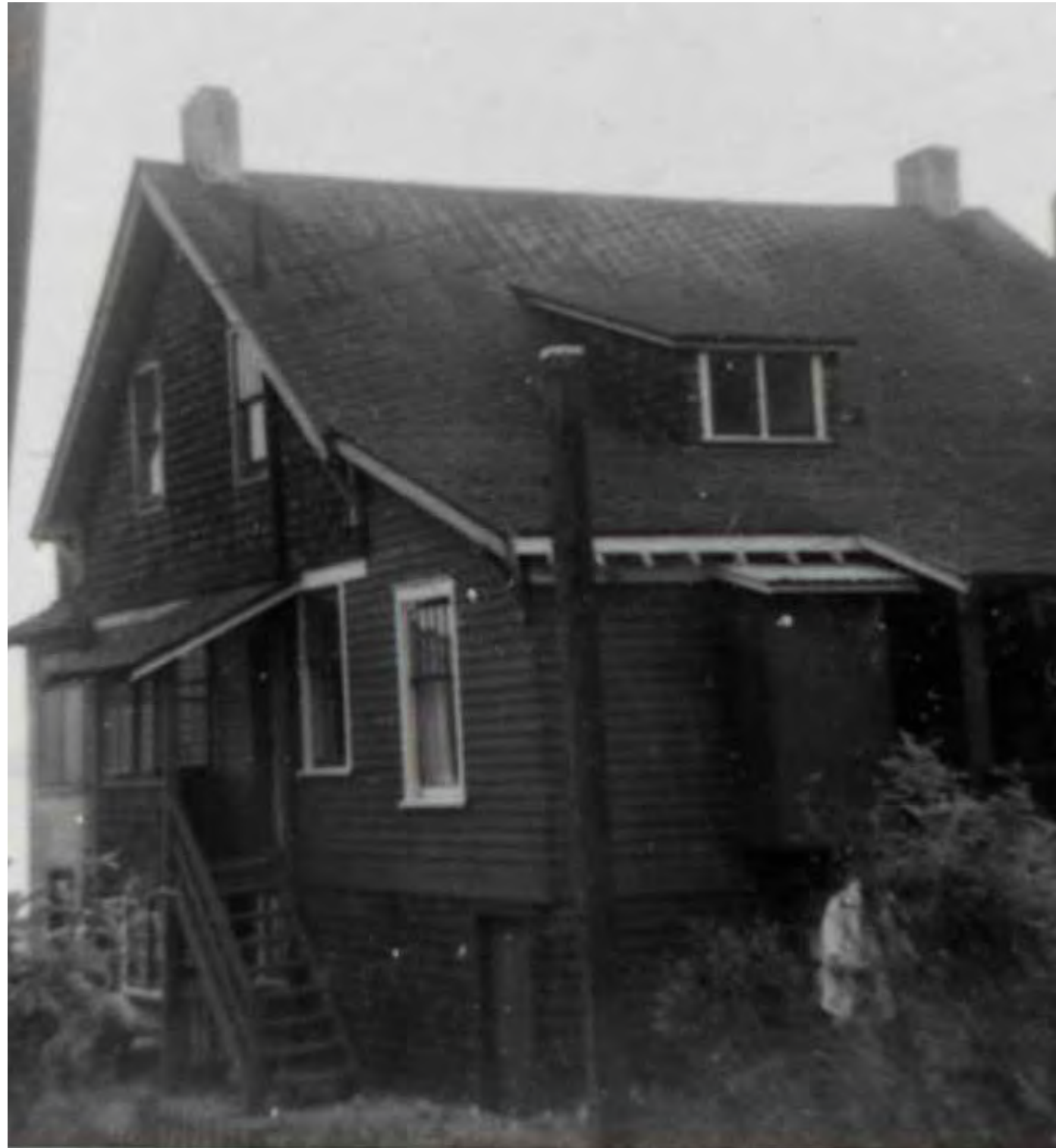
North Elevation facing Argyle Avenue. West Vancouver Archives 028.13.118.03.png
