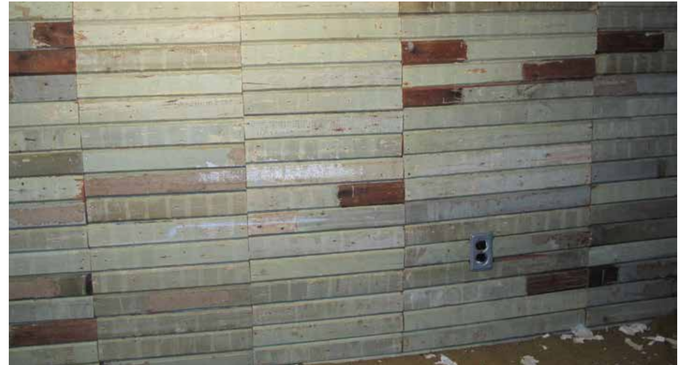
Basement Level wood sidings repurposed as cladding
