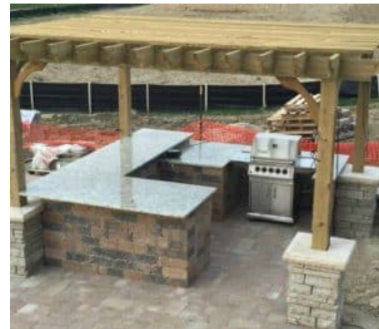
PERGOLA OVER KITCHEN AREA. TO BE GREY GRANITE COUNTER WITH BASALT STONE FACING
