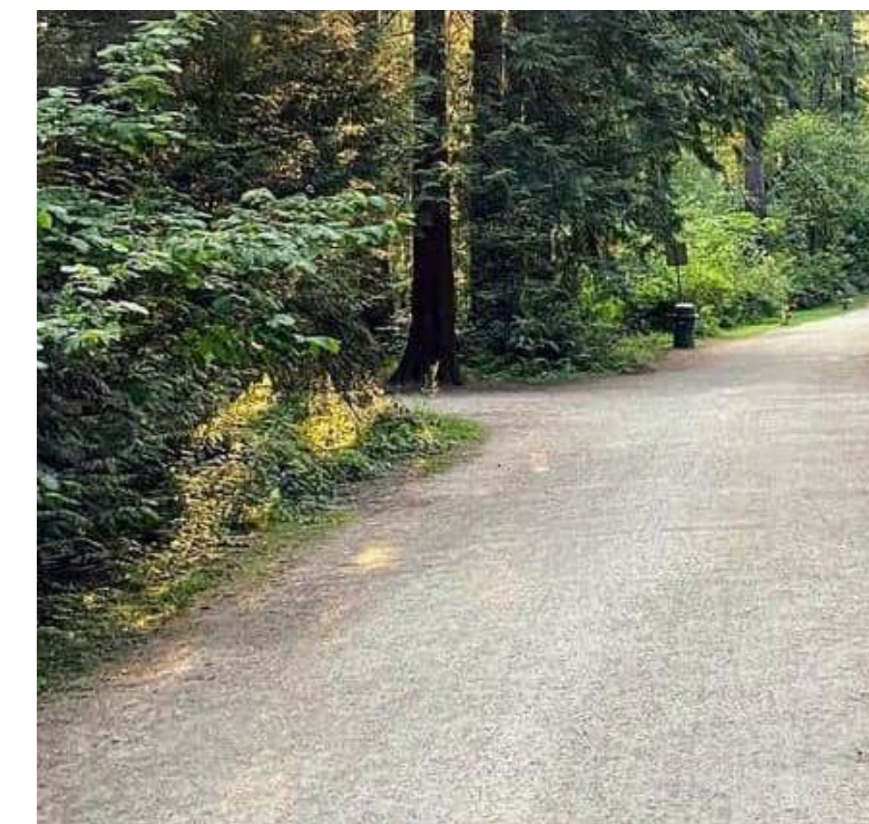
Compacted gravel at rear yard exit walkway
