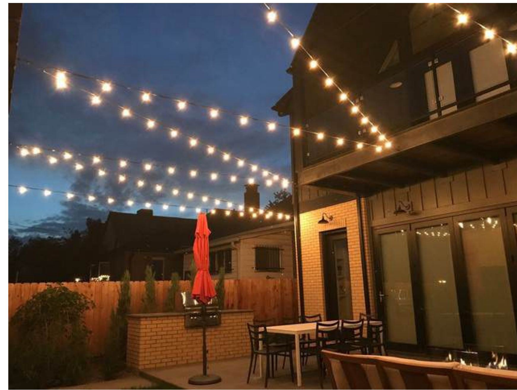
Catenary Lighting over rear yard deck
