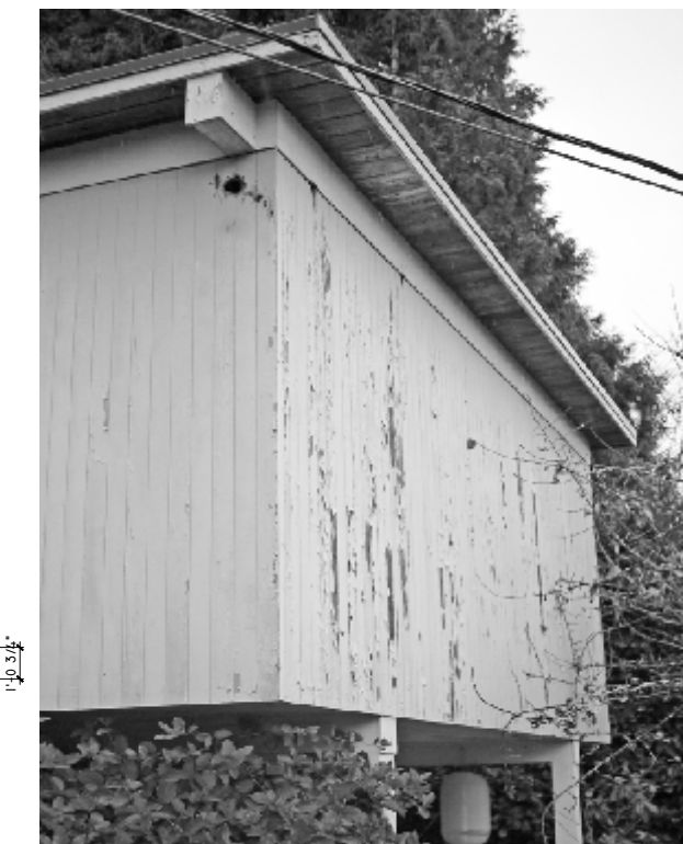
View of Existing Garage from Garden
