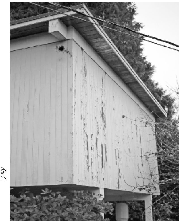
View of Existing Garage from Garden
