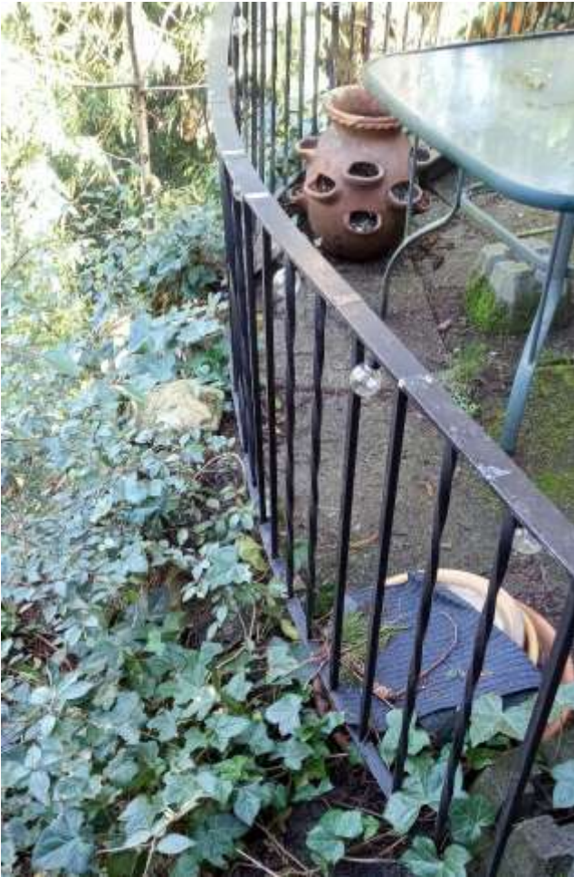
Figure 82: Original steel railing around north side terrace
