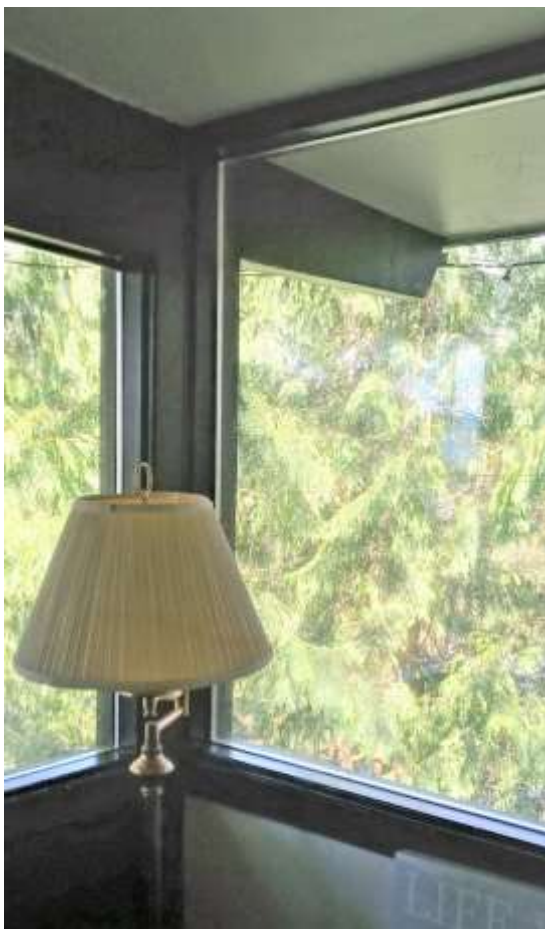
Figure 92: Exposed rafters projecting to the outside
