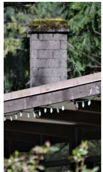
Figure 107: Chimney shaft facing east
