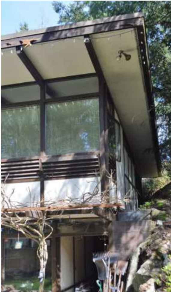
Figure 94: Southeast corner with roof overhang
