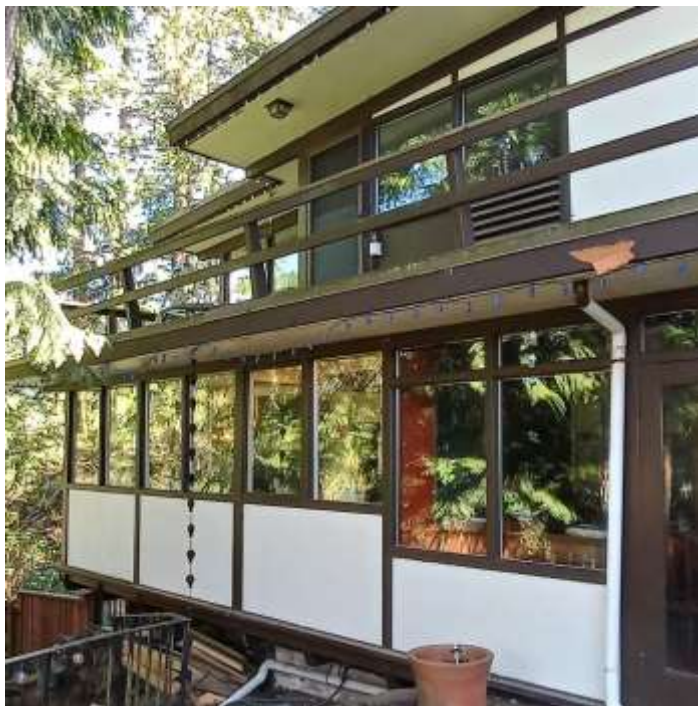
Figure 101: North side terrace
