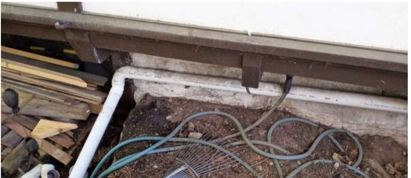
Figure 84: Concrete footing and drain pipe
