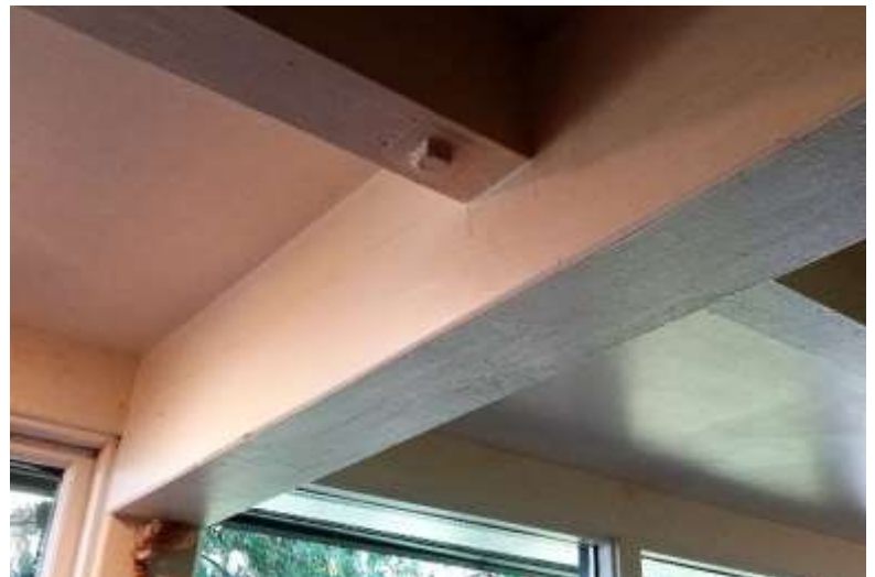
Figure 124: Steel structural member reinforcing the kitchen ceiling
