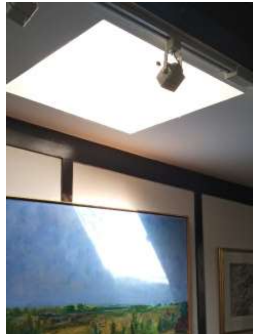
Figure 129: Second floor hall skylight
