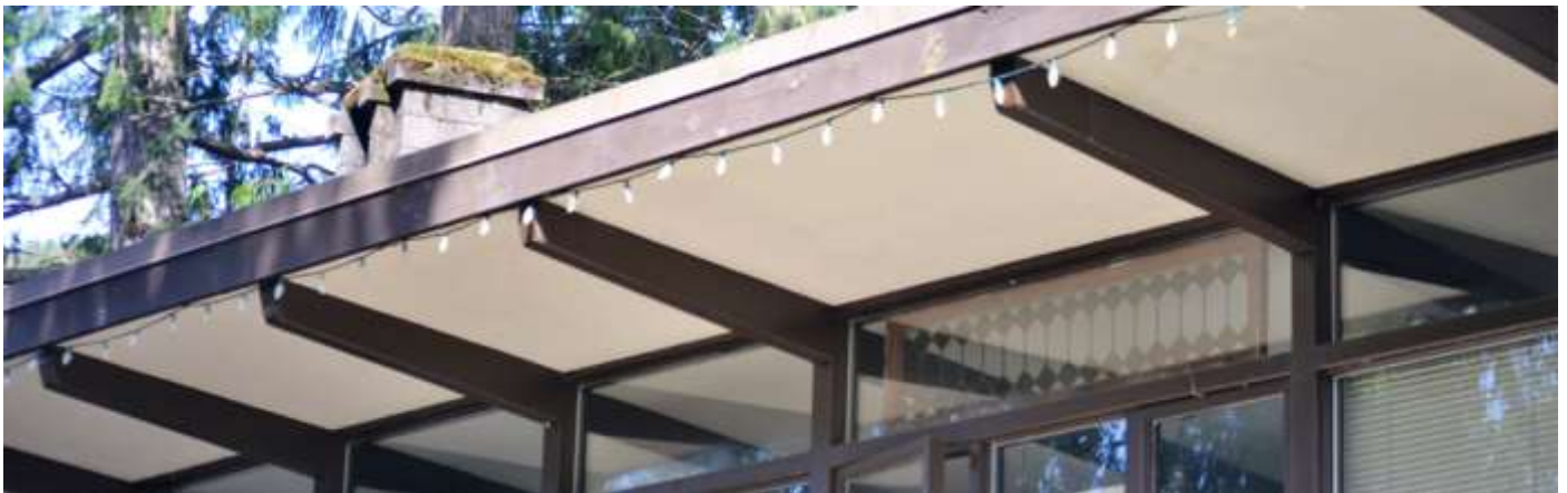
Figure 88: Roof overhang with exposed rafters
