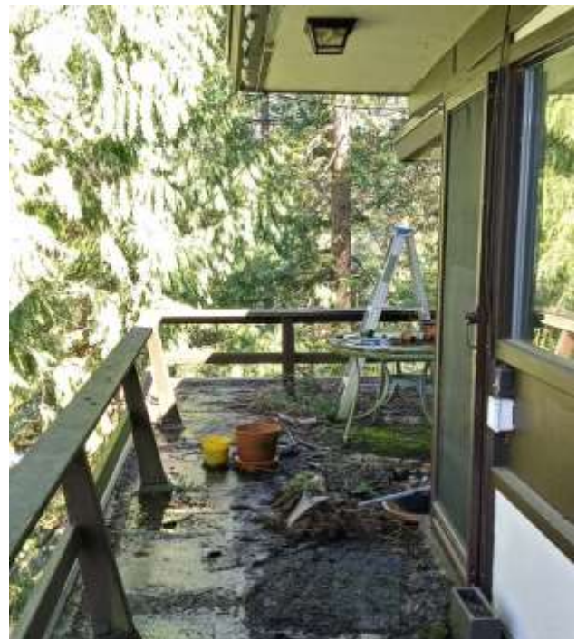
Figure 102: Second floor balcony
