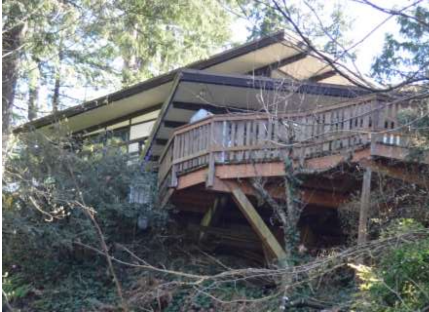
Figure 85: Original deck with 1970's extension on the right
