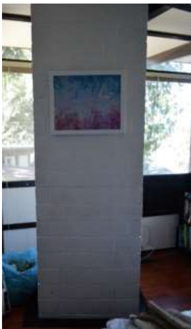
Figure 105: Chimney shaft through bedroom
