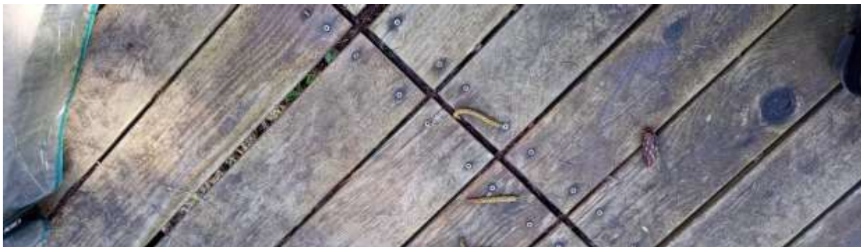
Figure 81: Wooden board deck floor
