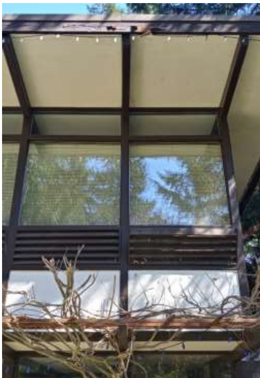
Figure 89: Roof overhang with exposed rafters
