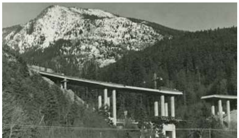
Figure 32: 1973 Nelson Creek Bridge view from the Eagle Harbour - 2166.WVA.RAH
