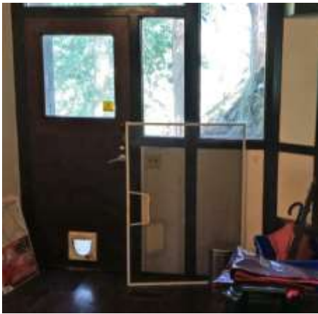
Figure 120: Storage door and window WE 03 -04
