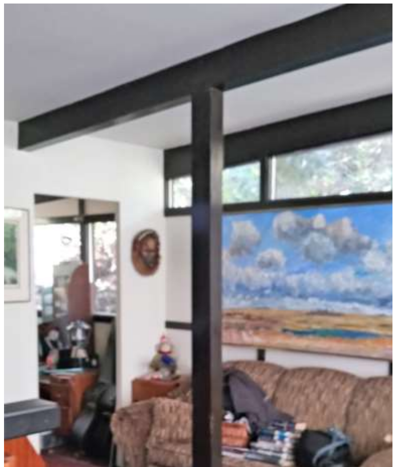
Figure 93: Free standing post supporting rafters
