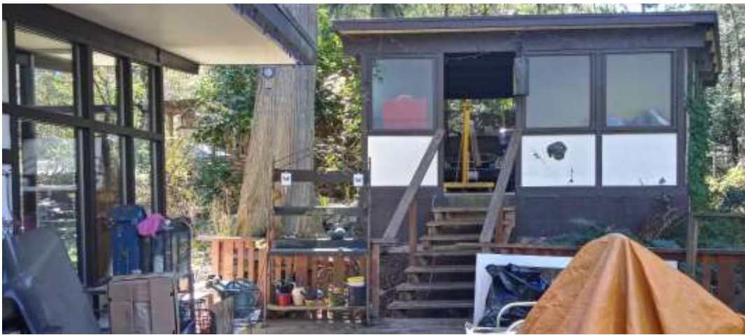
Figure 18: North elevation of car port from deck with southwest corner of main house on the left
