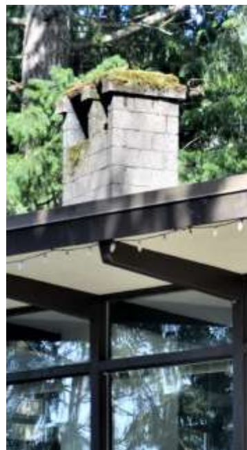
Figure 106: Chimney shaft facing south
