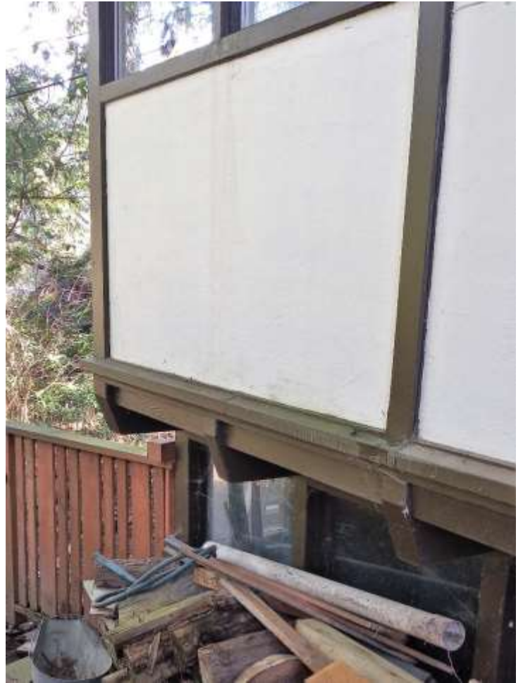
Figure 83: Crawl space under the east side of the house
