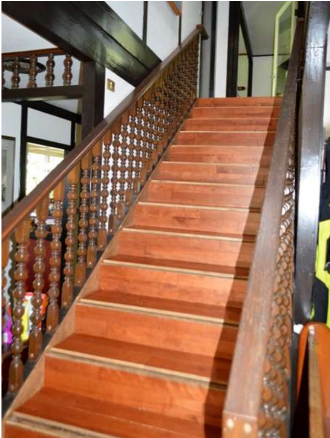
Figure 125: Main stair balustrade
