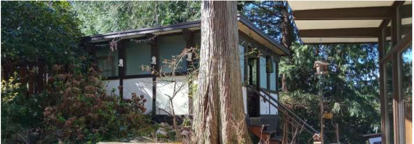
Figure 72: 1984 Car port / garage facing top of Larson Place in front of the house with access door from deck
