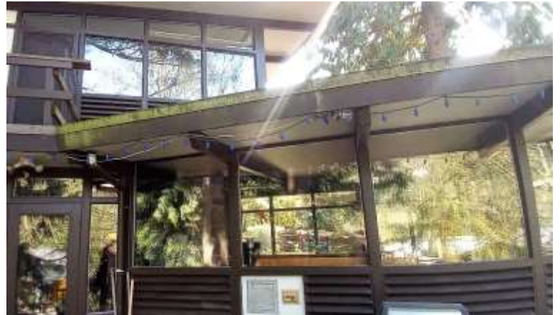
Figure 17: North elevation of living room wing
