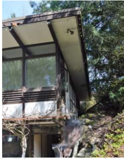
Figure 79: Stone embankment on the east side of the house
