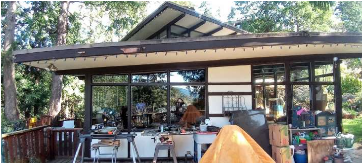
Figure 14: West elevation of the living room wing with main house beyond
