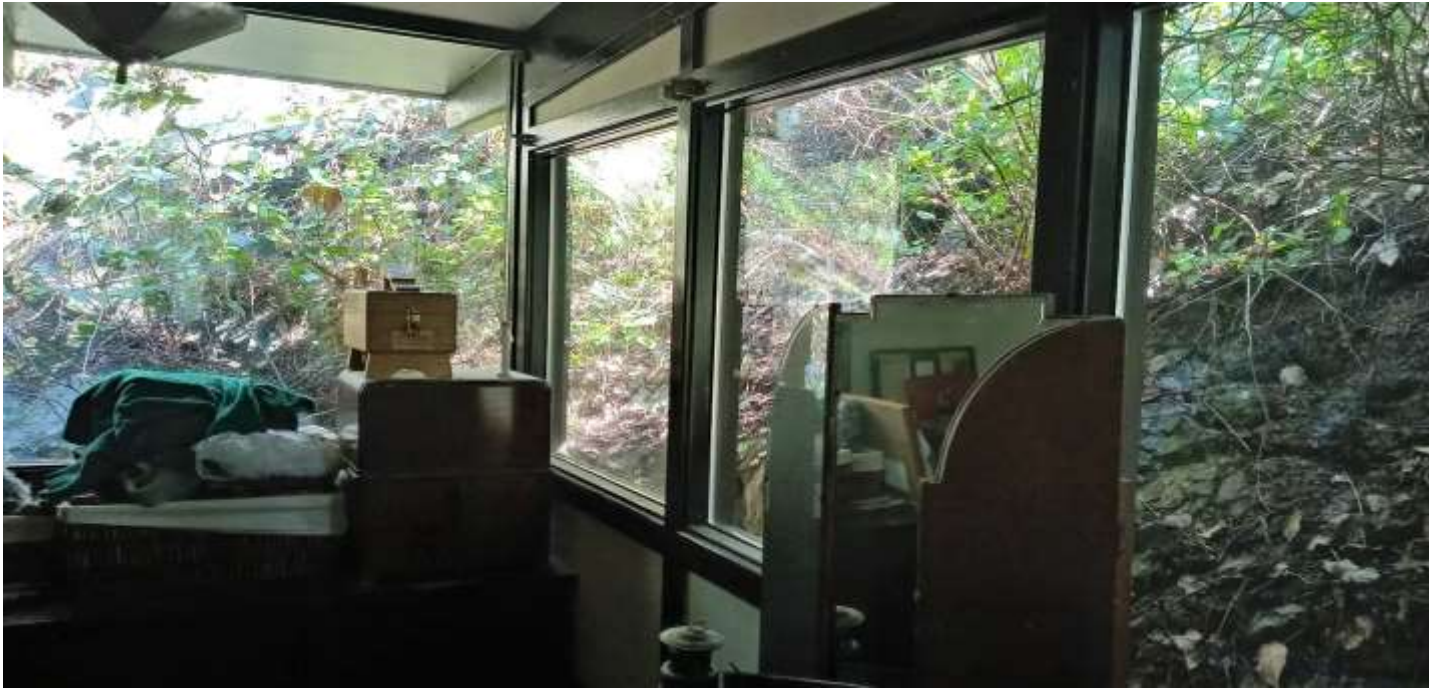
Figure 27: View of east embankment from lower floor family room
