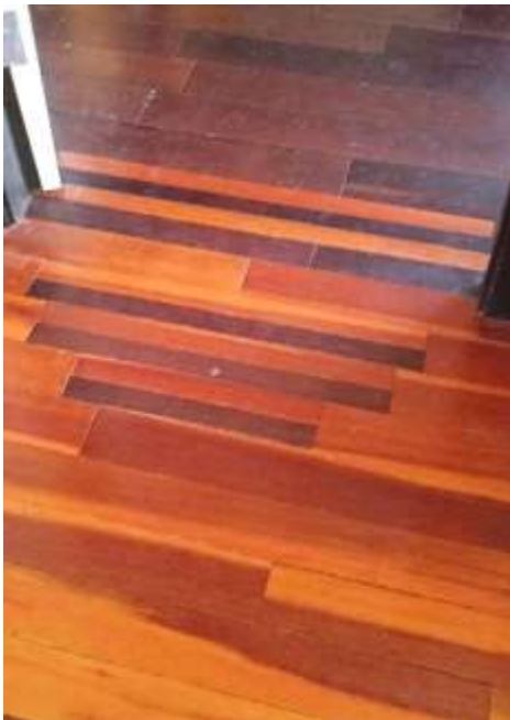
Figure 127: New wood floor
