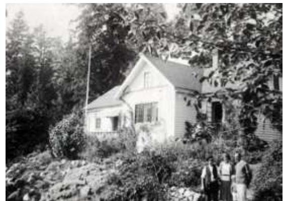
Figure 39: 1932 Caulfeild first house - 011.WVA.CAU
