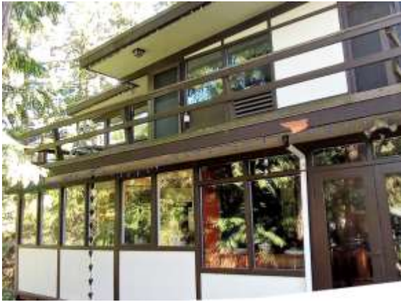
Figure 16: Northwest elevation of main house
