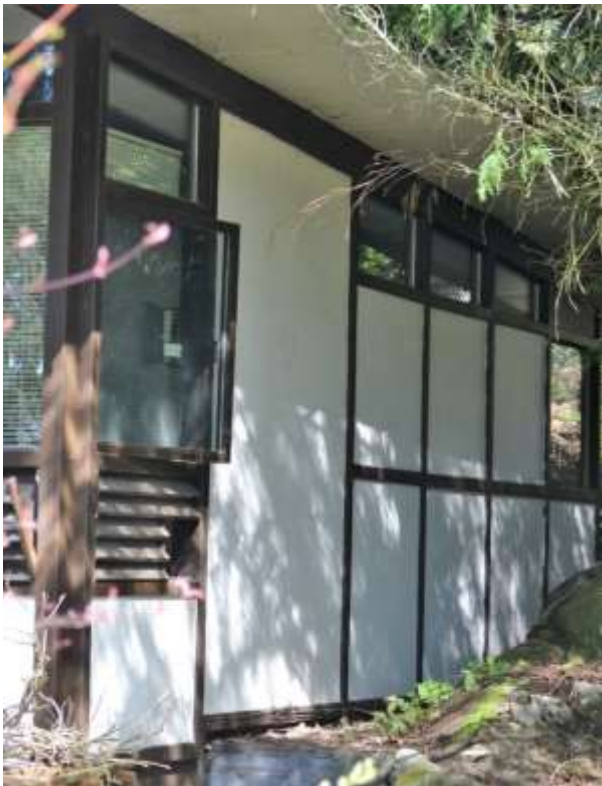
Figure 98: Exterior wall panels
