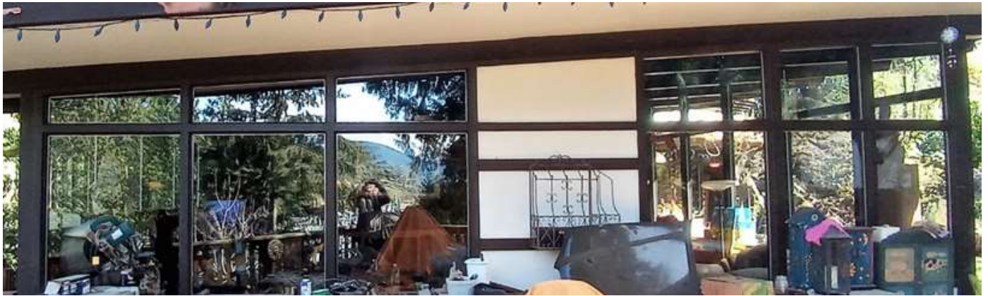
Figure 115: West side windows with transom WW 01 – WW 06
