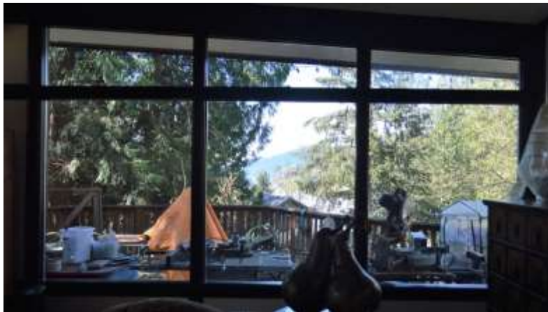
Figure 116: Living Room windows with transom WW 01 – WW 03
