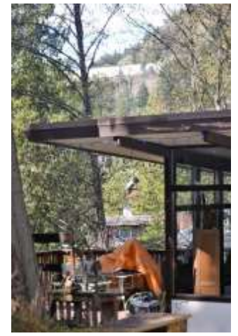
Figure 19: North view of deck
