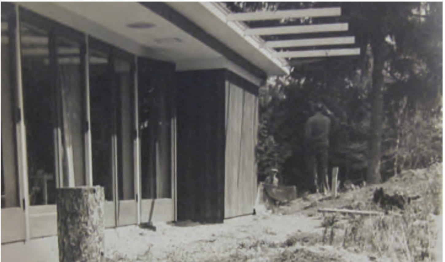
Construction image, showing Bertie, Lacey (dog) and the construction of the exterior yard, ca. 1940s, Vancouver Art Gallery Archives
