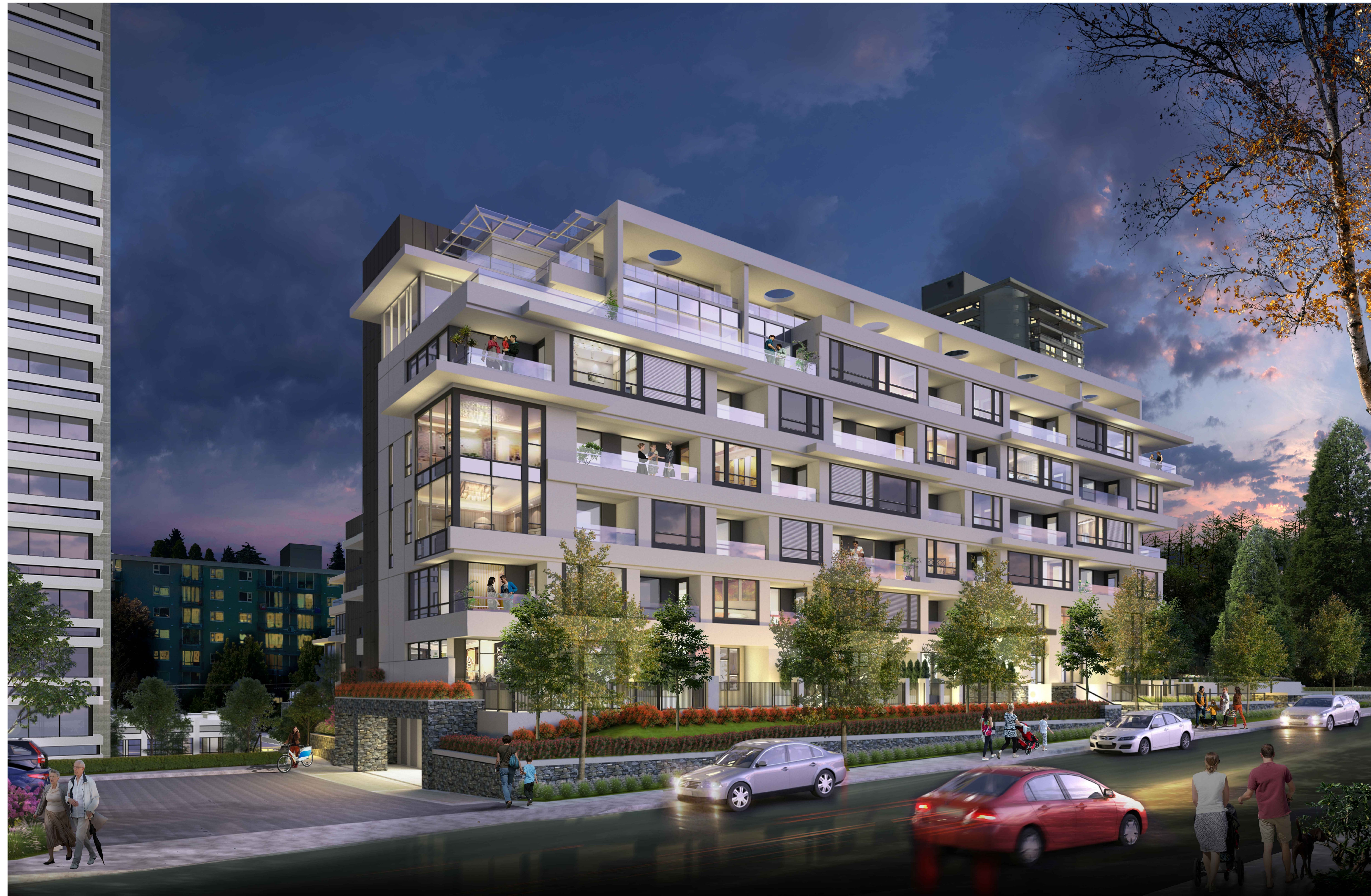
1 Bldg. 1 (View from NE along Esquimalt Ave.)
