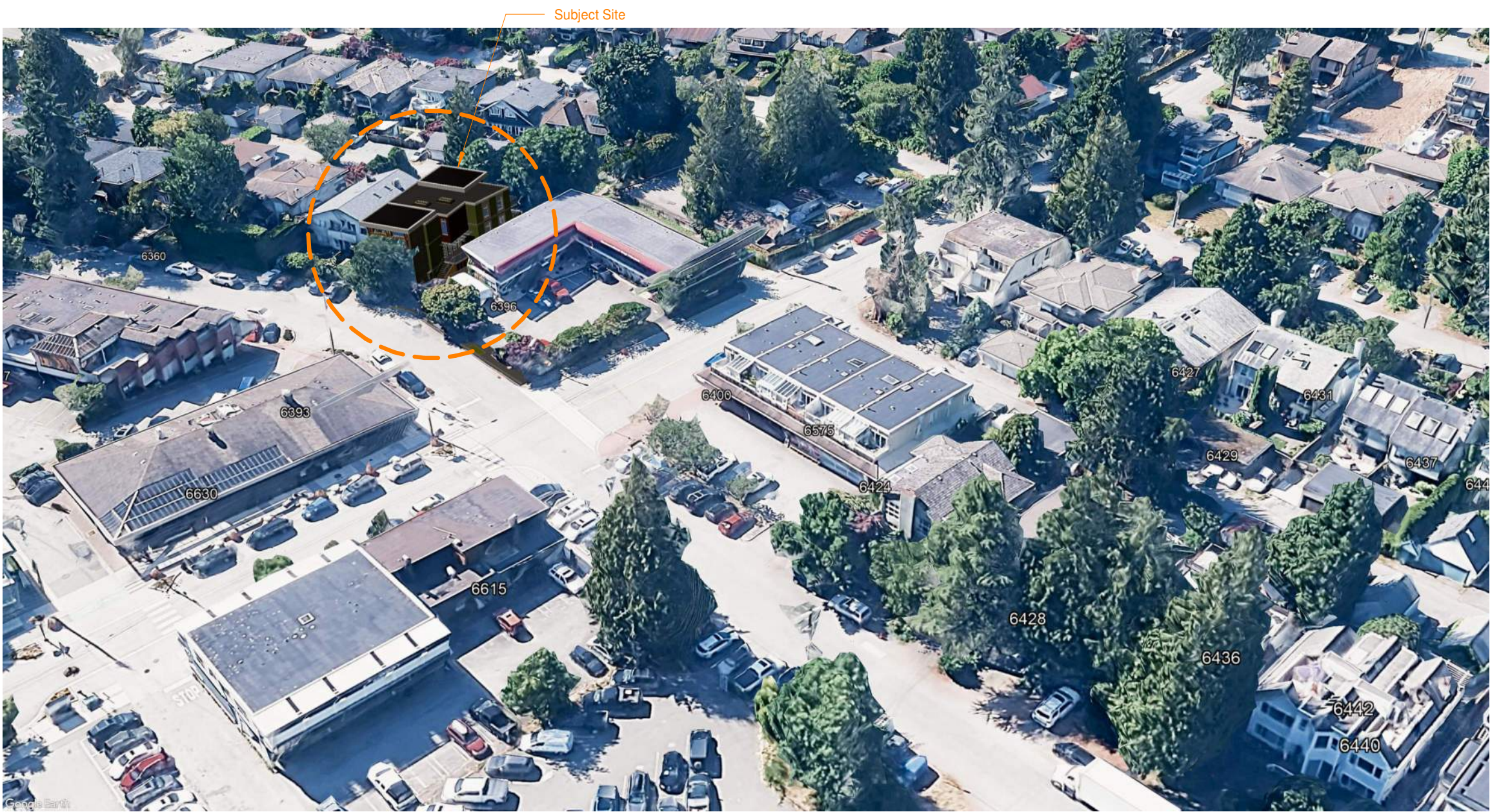
AERIAL VIEW OF SITE FROM BRUCE STREET
