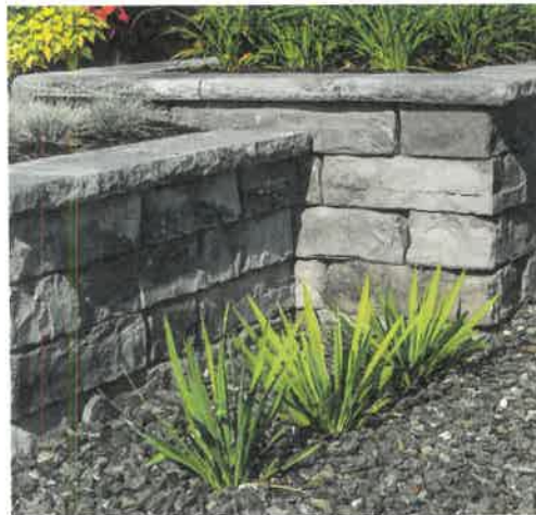
Rosetta Kodah - stone faced retaining wall
