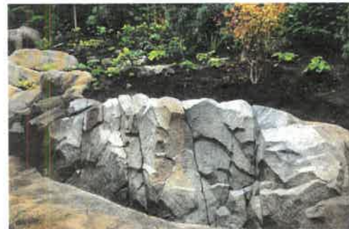
Cast in Place - Shotcrete Feature Wall
