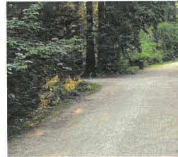
Compacted gravel at rear yard exit walkway
