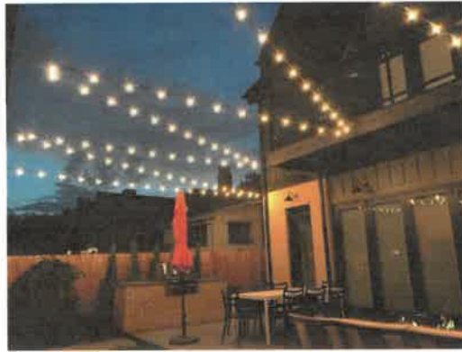
Catenary Lighting over rear yard deck
