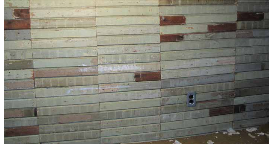
Basement Level wood sidings repurposed as cladding
