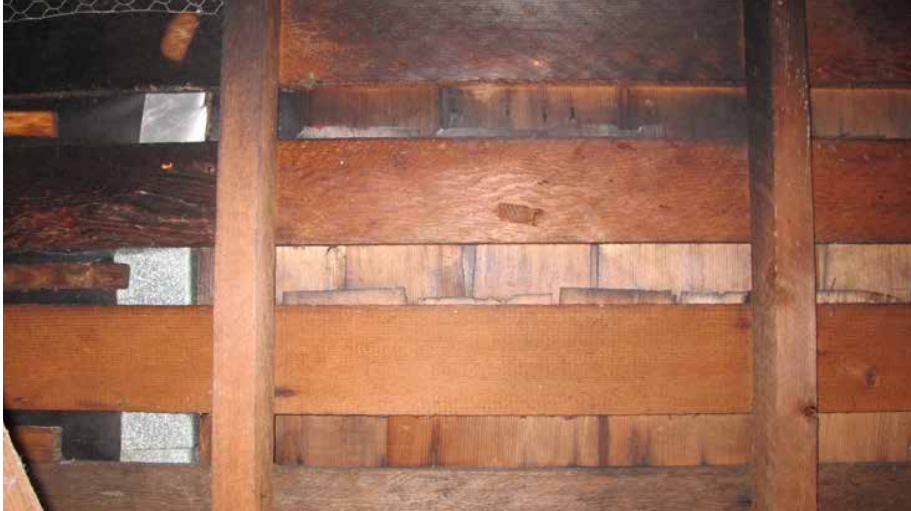
Underside of intact cedar shingle roofing
