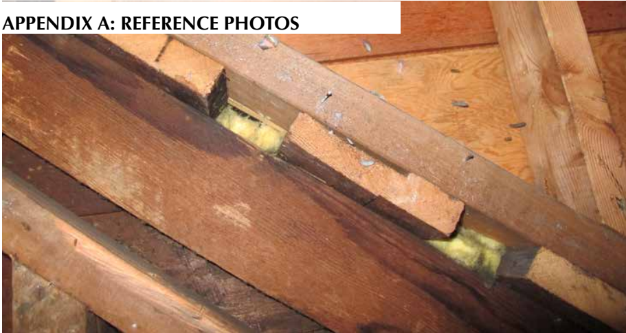
Cut-through roof structure showing original nailing strips.
