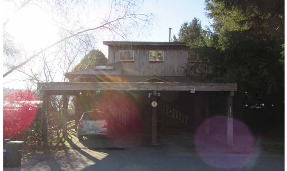
Existing North Elevation. January 2017
