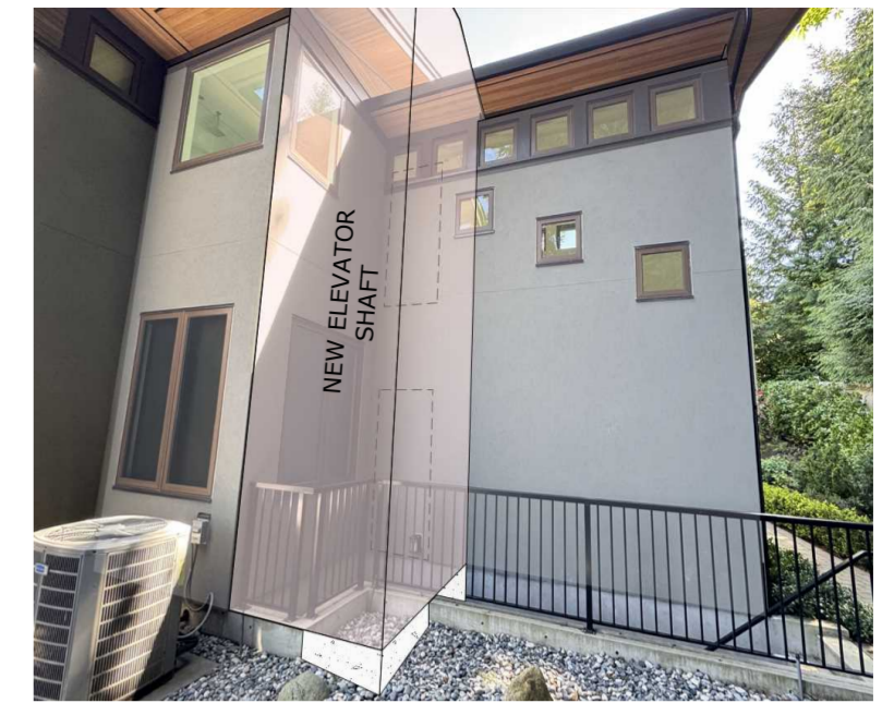
ELEVATOR SHAFT PHOTO OVERLAY
