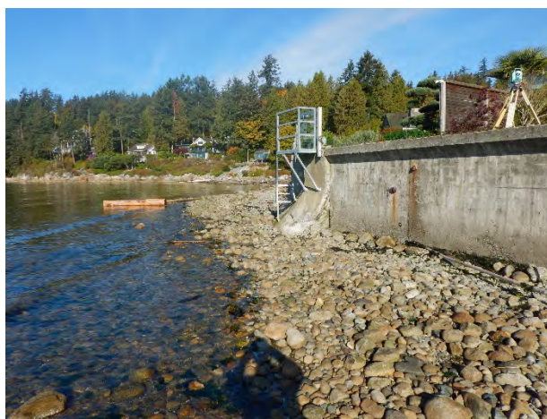
Photo 4. Potential scour near the wall, looking east of the property
