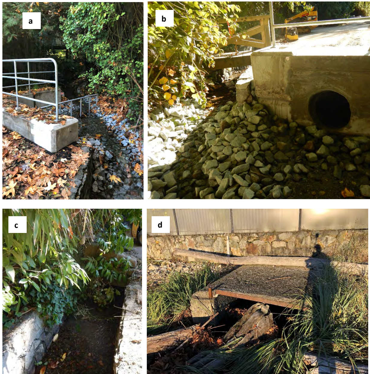
Figure B.3. Claymore Creek inlet and outlet photos (a: Claymore Creek at Ross Crescent, b: culvert inlet, c: constructed channel, d: debris at crossing outlet)
