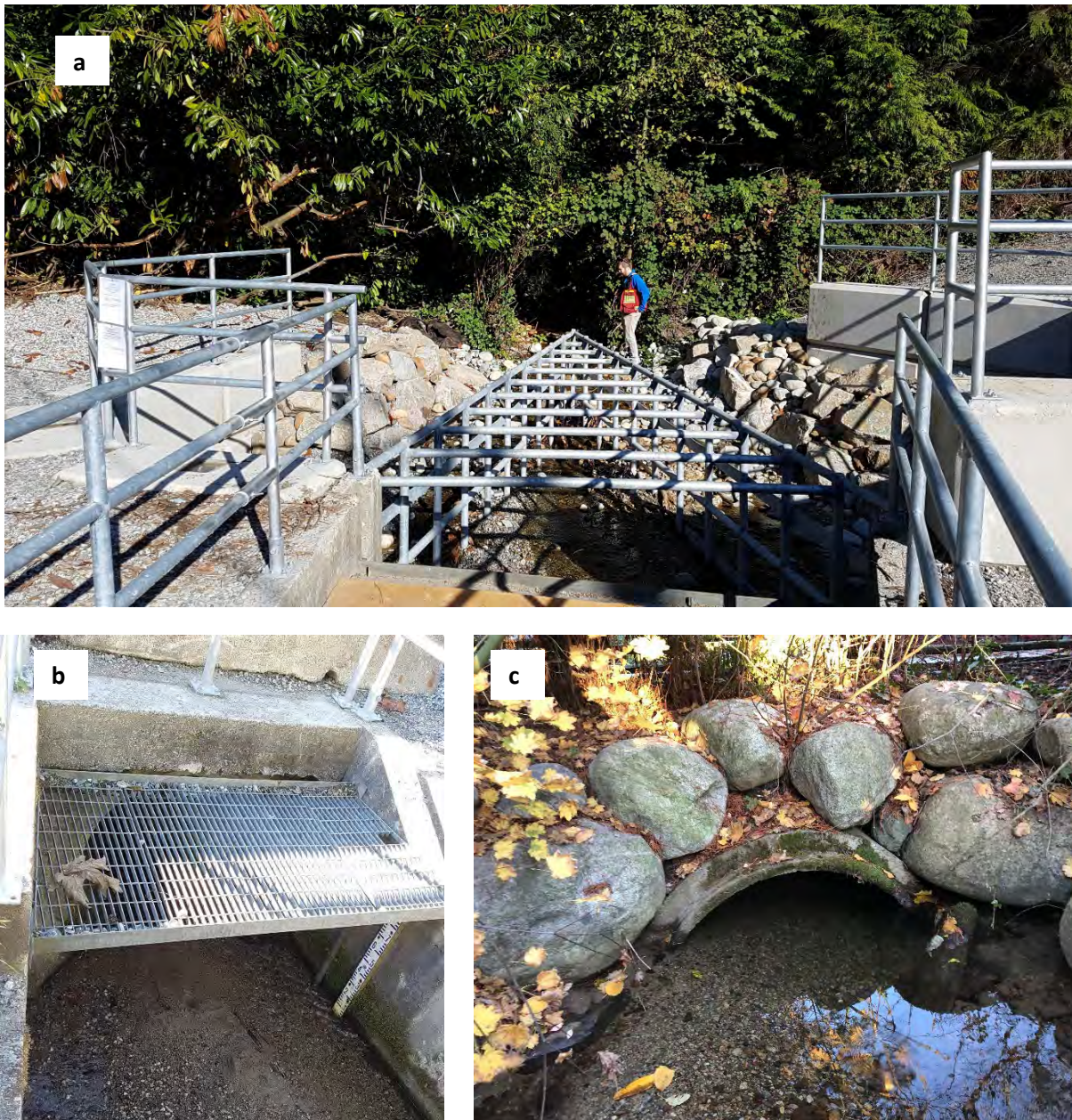
Figure B.2. Willow Creek photos (a: new trash rack at inlet, b: culvert inlet, c: outlet)
