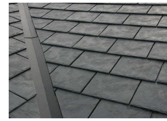
SLATE SHINGLES ROOF
