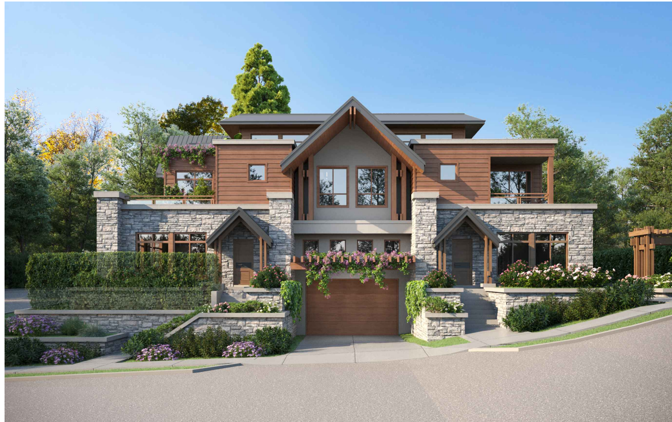
VIEW FROM 29TH STREET
