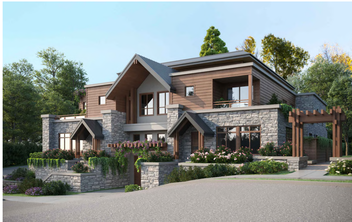
VIEW FROM 29TH STREET (NORTH EAST)
