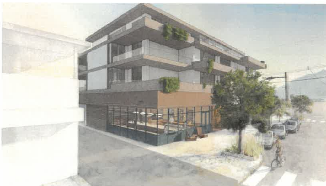
View From Royal Ave Looking North West
