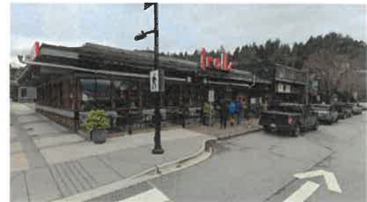
3 | NE CORNER OF SITE
