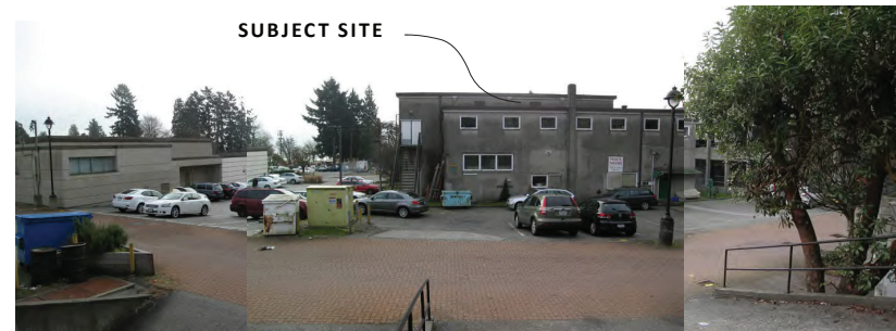
VIEW LOOKING SOUTH TOWARDS SUBJECT SITE
