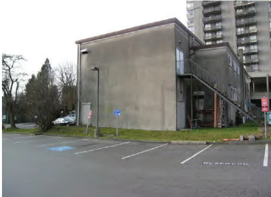
3- STREET VIEW: LOOKING EAST
