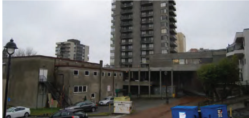
4- STREET VIEW: LOOKING SOUTH-EAST
