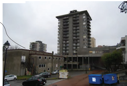
VIEW LOOKING WEST TOWARDS SUBJECT SITE
