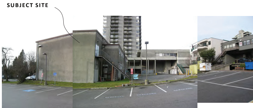
VIEW LOOKING WEST TOWARDS SUBJECT SITE
