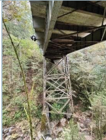
010. East Pier Abutment
