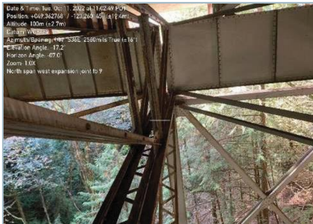
34. Vertical Bracing over Pier Section, Typ.
