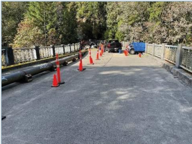
011. Bridge Deck Viewing West
