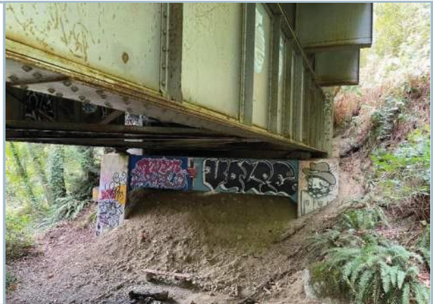
017. Jump Span Cap Beam at West Abutment
