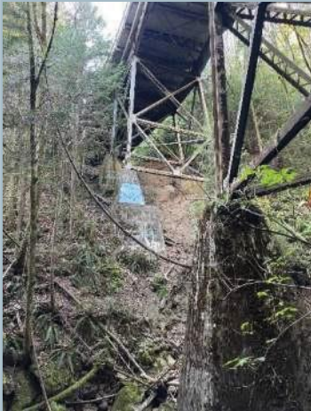
009. West Pier Abutment
