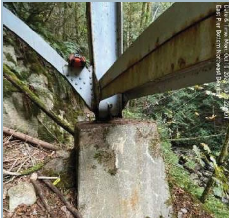
014. Northeast Pier Pedestal at West End
