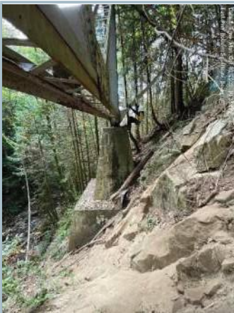
016. Southeast Pier Pedestal at West End
