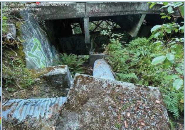
029. Stormwater Outfall at North Section of East
