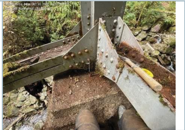
203. Pier Corner Connection, Typ.
