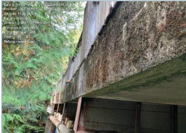
026. South Profile Parapet
