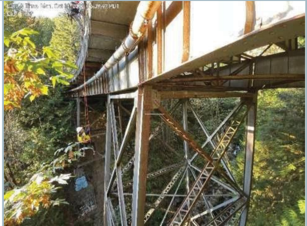
004. South Elevation (Note Existing Utility Pipe)
