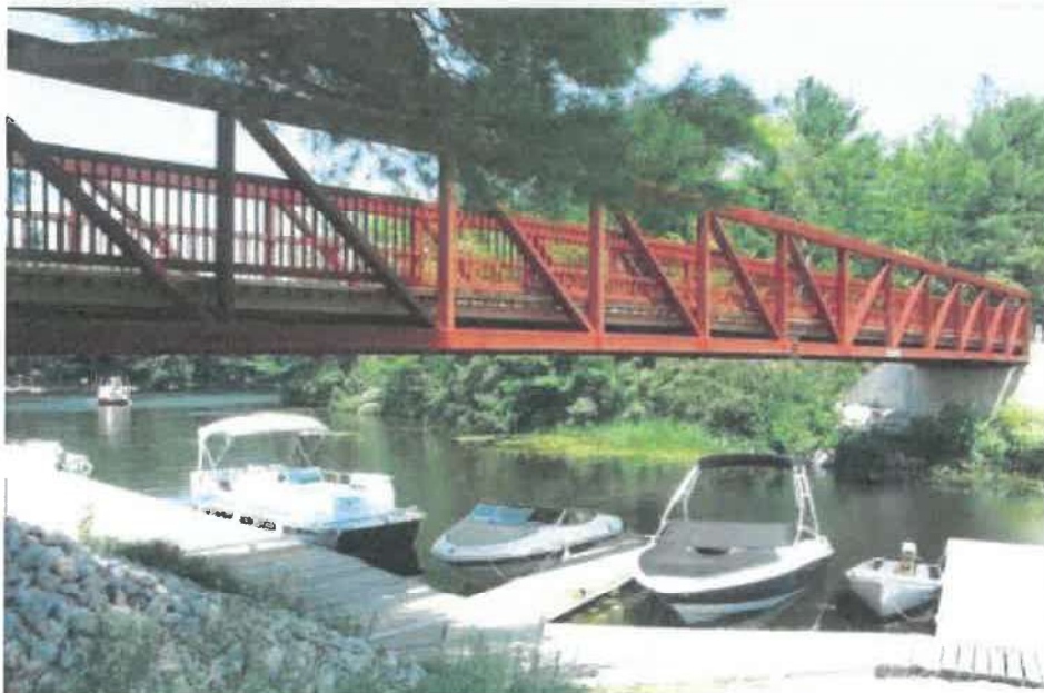
Figure 1 - Example of a Weathering Steel truss from Algonquin Bridge
