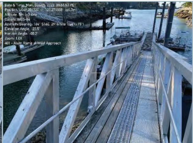
014. Aluminum Gangway Truss Rail, Typ.
