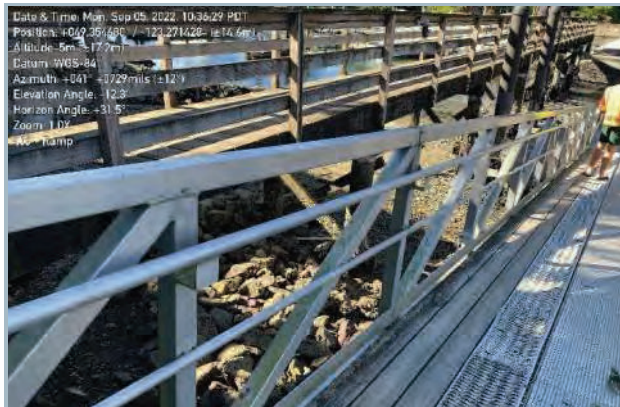
007. Gangway Railing & Truss Orientation
