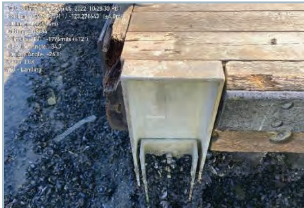
009. Dock Corner Restraint Connection, Typ.
