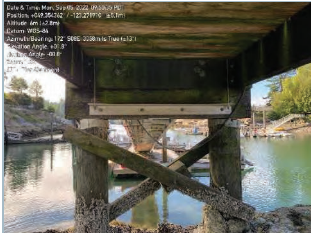
020. Gangway Access Platform to Timber Pier Connection
