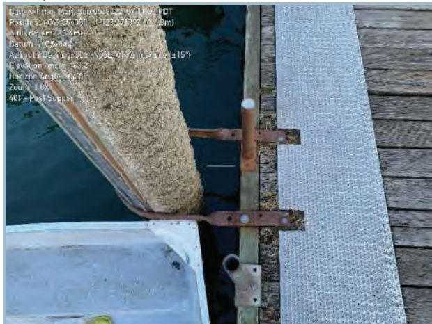
034. Dissimilar Timber Pile Restraint
