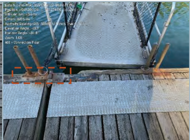
035. Overlapping Plates at Dock Connection
