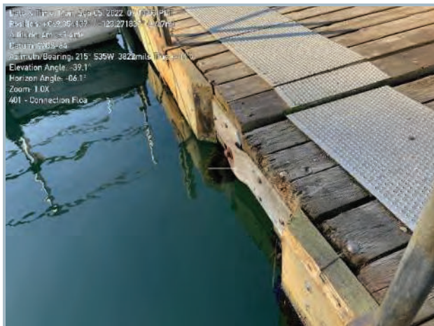
022. Anchored Plate Dock Connection
