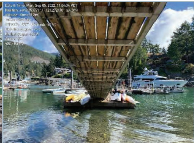
012. East Segment Gangway Soffit
