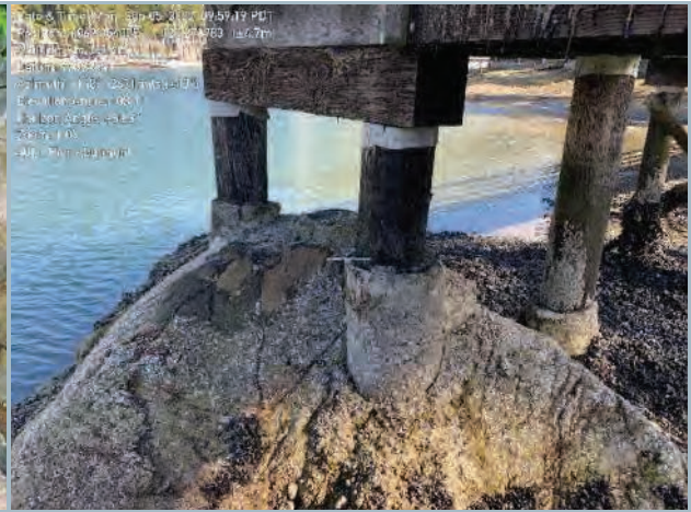
008. West Pier Abutment on Concrete Pedestal and Bedrock
