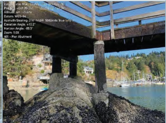
010. West Pier Abutment on Bedrock
