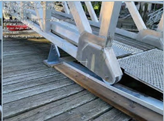
016. Gangway Slider Connection Mechanism
