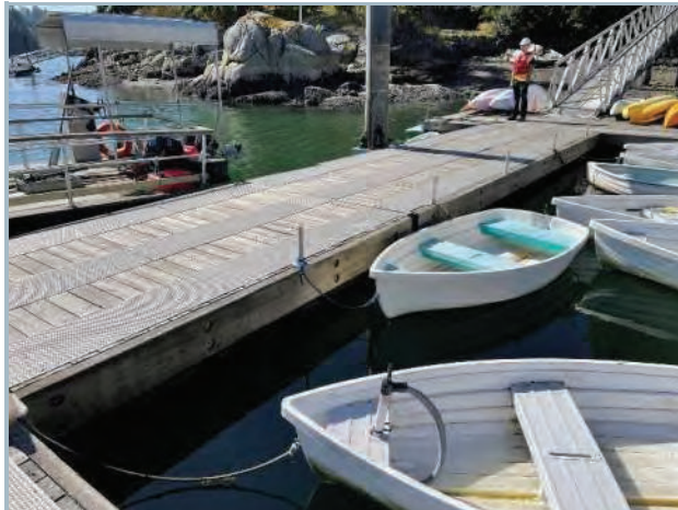
009. Deck of East Intermediate Landing Dock
