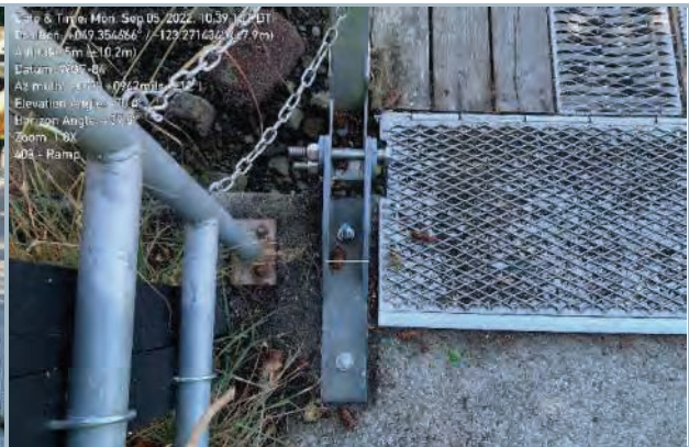
008. Gangway Connection to East Abutment
