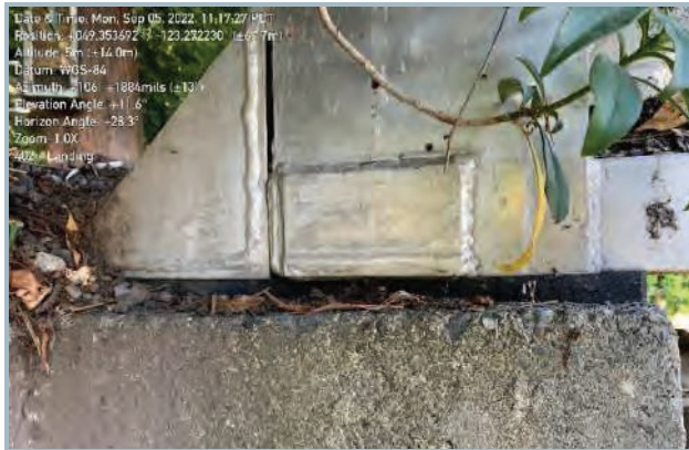
015. Shear Key at Abutment
