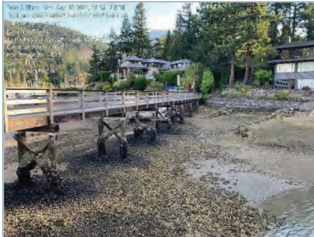
009. Braced Timber Piers, Typ.
