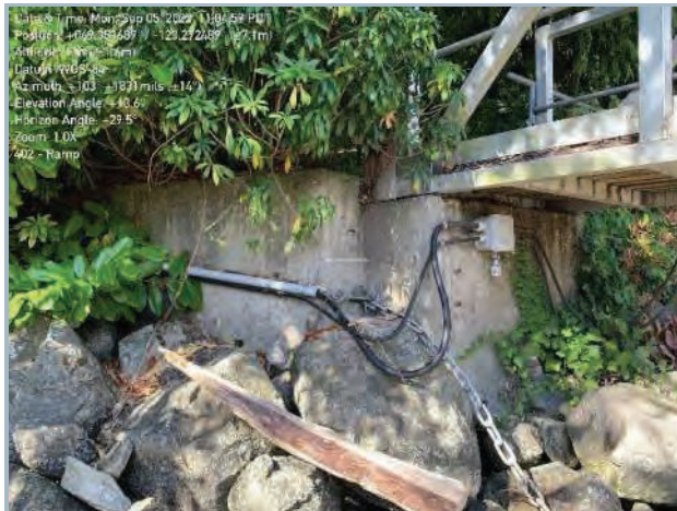
007. Southwest Abutment Wingwall
