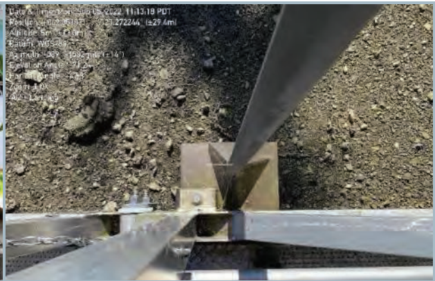
016. Anchored Pier Connection with Elastomer Bearing
