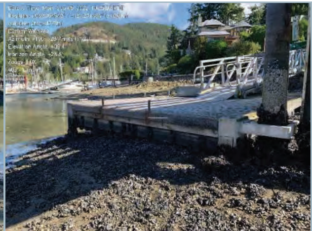
002. West Elevation (Note Connection to Timber Pile at Southwest)
