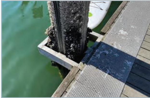
013. Exterior Dock-Timber Pile Restraint Connection, Typ.
