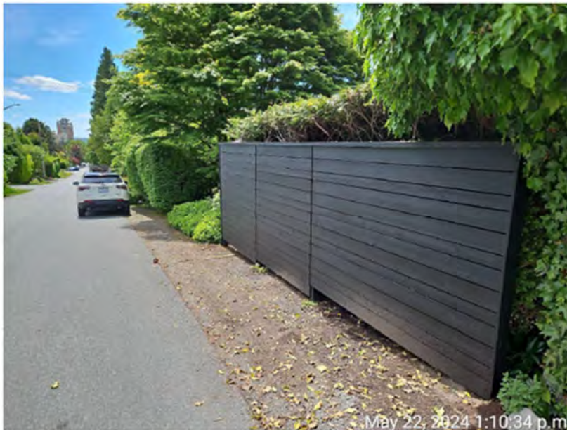
Figure 1: Current Fence Condition
