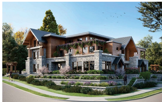
Corner View: Marine Drive & 29 th Street
