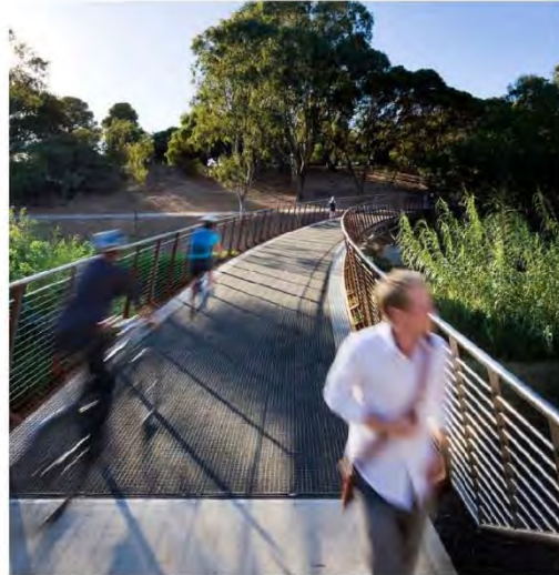
River Torrens Bridge, Australia
