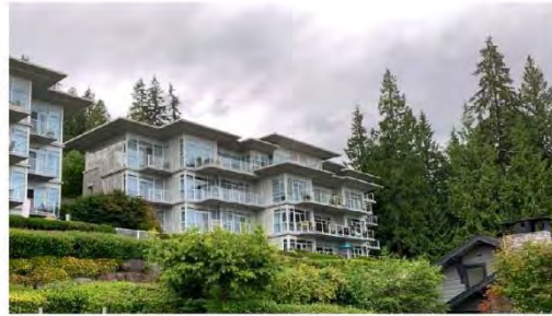
Boulders, West Vancouver
