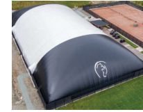
COMPONENT: EXTERNAL FINISH MATERIAL: TEDLAR PVF FILM COLOUR: VARIES
