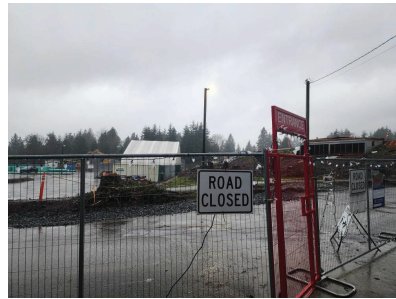
EXISTING PARKING LOOKING WEST
