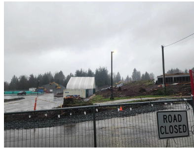
EXISTING PARKING LOOKING WEST
