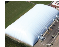
COMPONENT: EXTERNAL FINISH MATERIAL: TEDLAR 10% TRANSLUCENT PVF FILM COLOUR: EGG-SHELL
