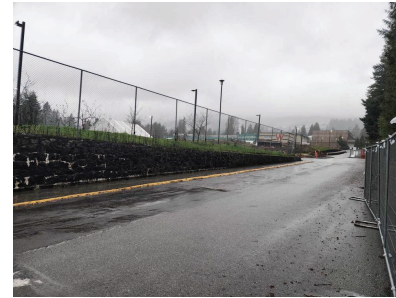
EXISTING TRACK LOOKING NORTHWEST
