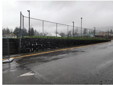
EXISTING TRACK LOOKING NORTHWEST
