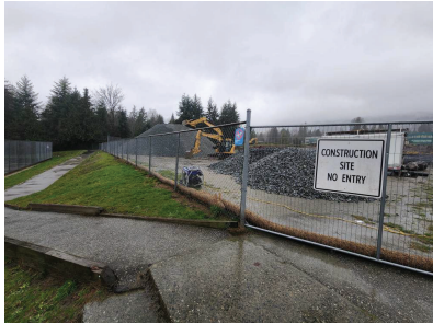
EXISTING PATH LOOKING SOUTHWEST
