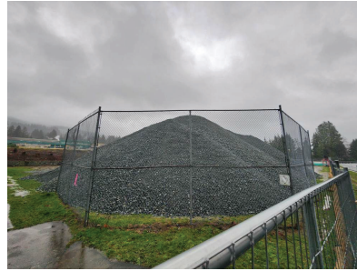
EXISTING SITE LOOKING NORTHEAST
