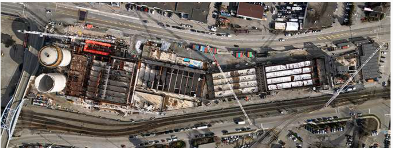
Aerial view of the North Shore Wastewater Treatment Plant construction site
