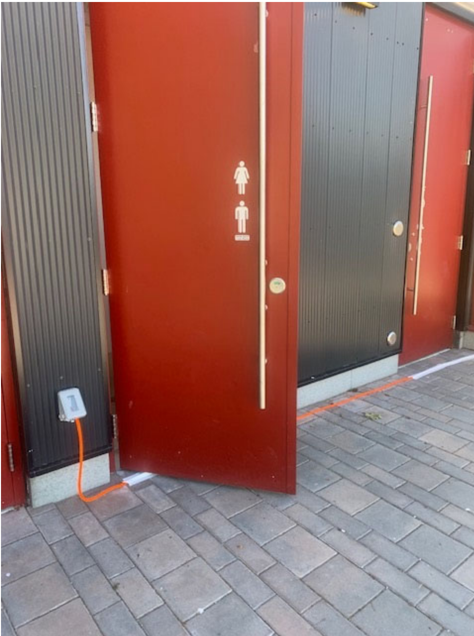
Electrical cord continued across a major entry sidewalk
