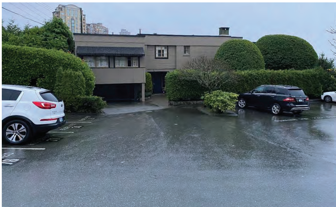
Figure 3-4. Existing dwelling western access and neighboring parking lot – facing east.
