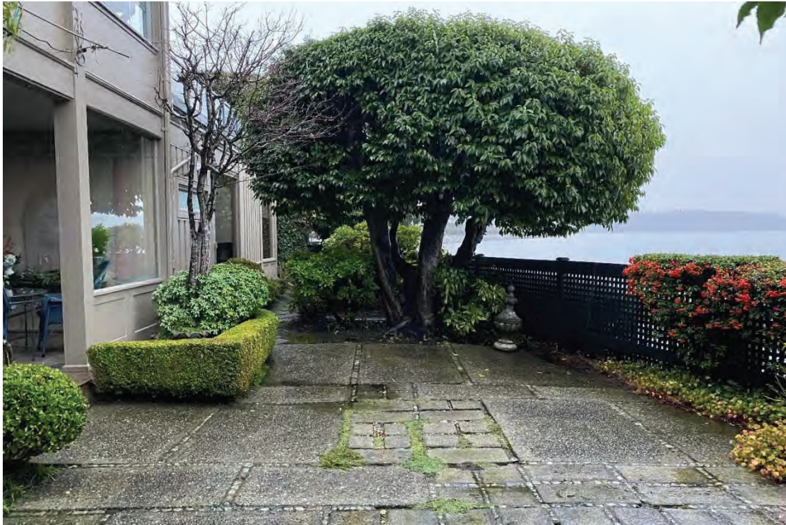
Figure 3-5. Concrete patio illustrating the setback between existing dwelling and Centennial seawalk – facing east.
