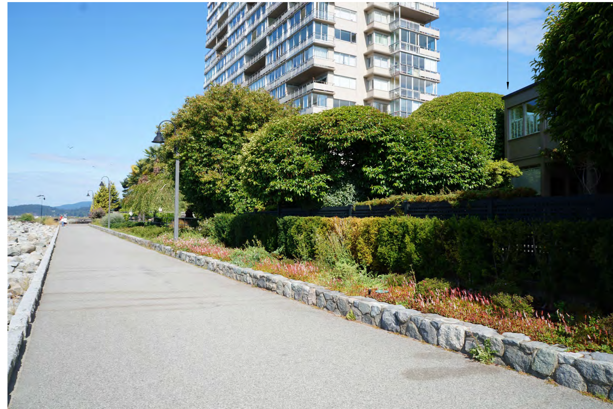
VIEW OF EXISTING HOUSE + SEASTRAND BUILDING FROM SEAWALK
