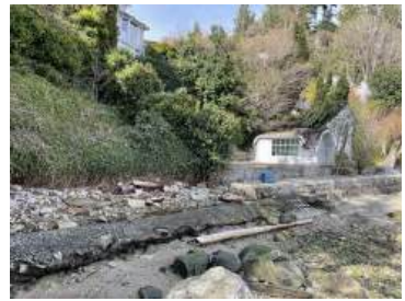
VIEW LOOKING NORTH THIS VIEW SHOWS THE EXISTING POOL HOUSE AND OTHER HARDSCAPE TERRACES ENCRDACHING INTO THE FORESHORE. THEY ARE PROPOSED TO BE REMOVED IN THE NEW DESIGN WITH ADDED SOFT COVERAGE OVER THE SEWER PIPE WHICH IS GETTING UNDERPINNED DUE TO EROSION.
