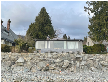
EXISTING ROCK WALL AT FORESHORE ALONG 2870 BELLEVUE
