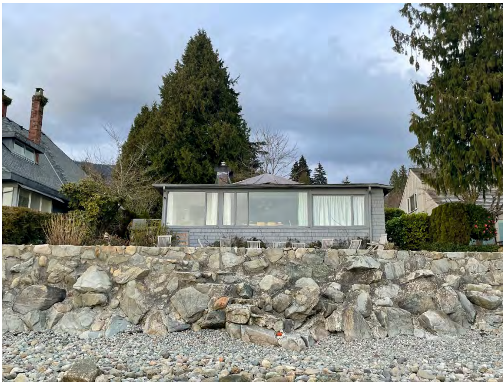
Figure 3 – Close-up view of the seawall and upper foreshore at the site (Lamoureux Architect)
