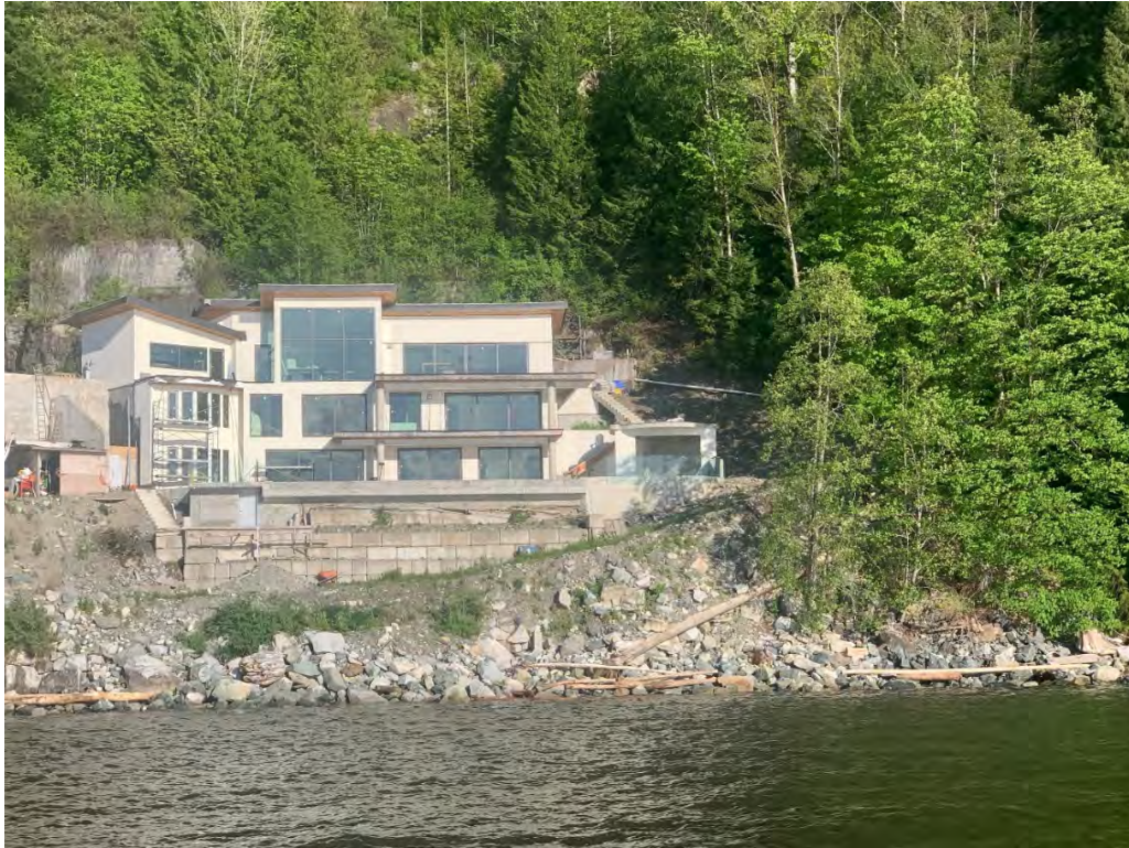
Figure 2 – View from Howe Sound (looking eastwards)
