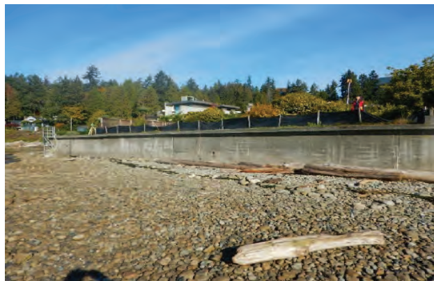
Figure 3 – Photograph of Foreshore Protection Wall
