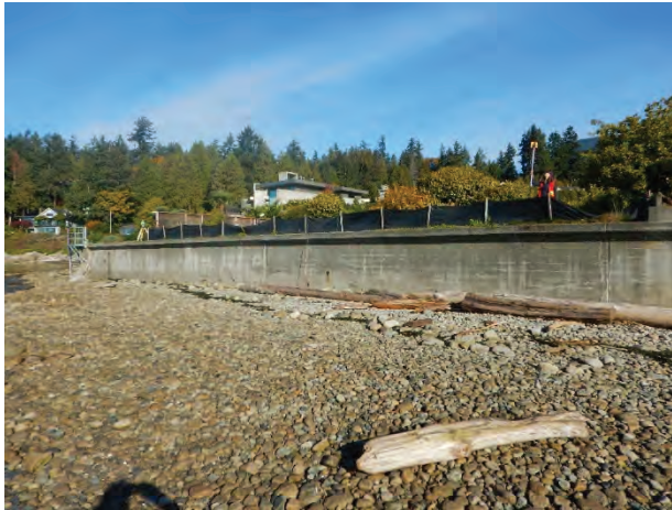
Photo 1. Towards site from beach
