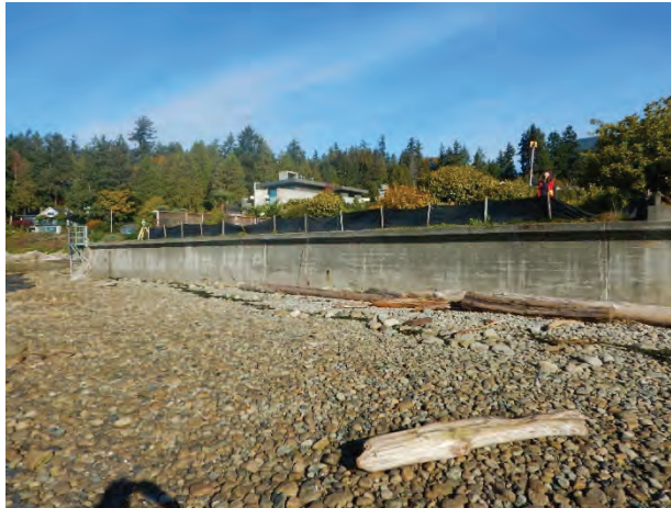
Photo 1. Towards site from beach
