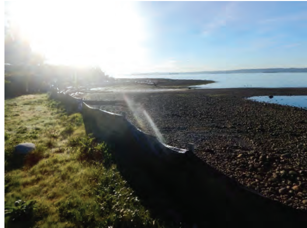
Photo 2. Southeast towards outlet of Willow Creek from top of concrete wall.
