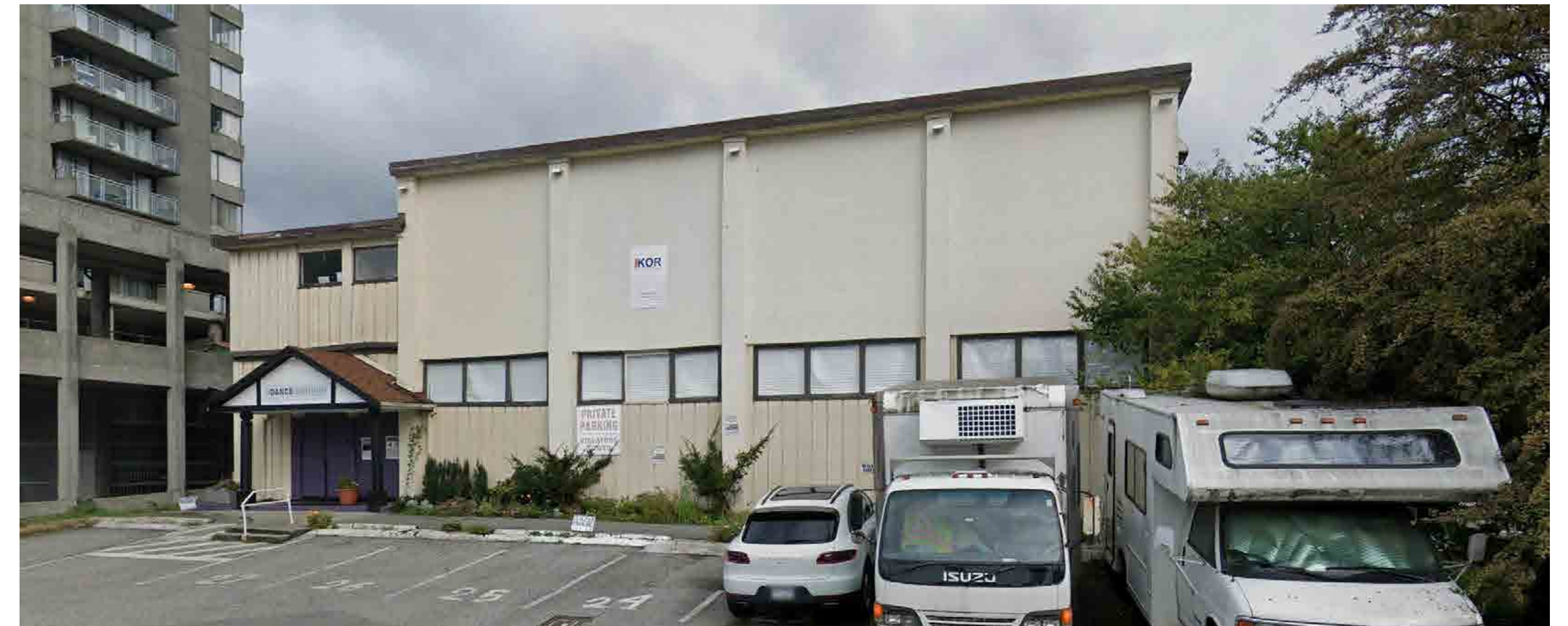
2- STREET VIEW: LOOKING NORTH-EAST
