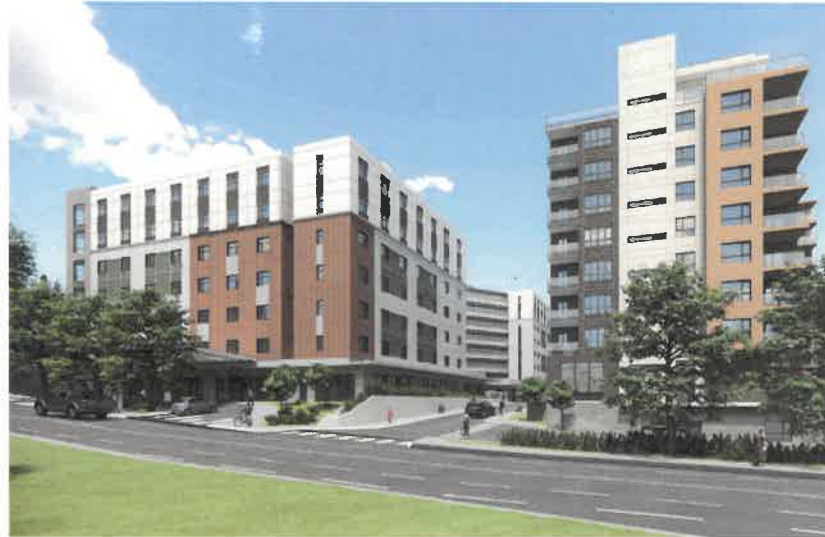
2 VIEW LONG TERM CARE ENTRY AND INDEPENDENT LIVING PARKING ACCESS
