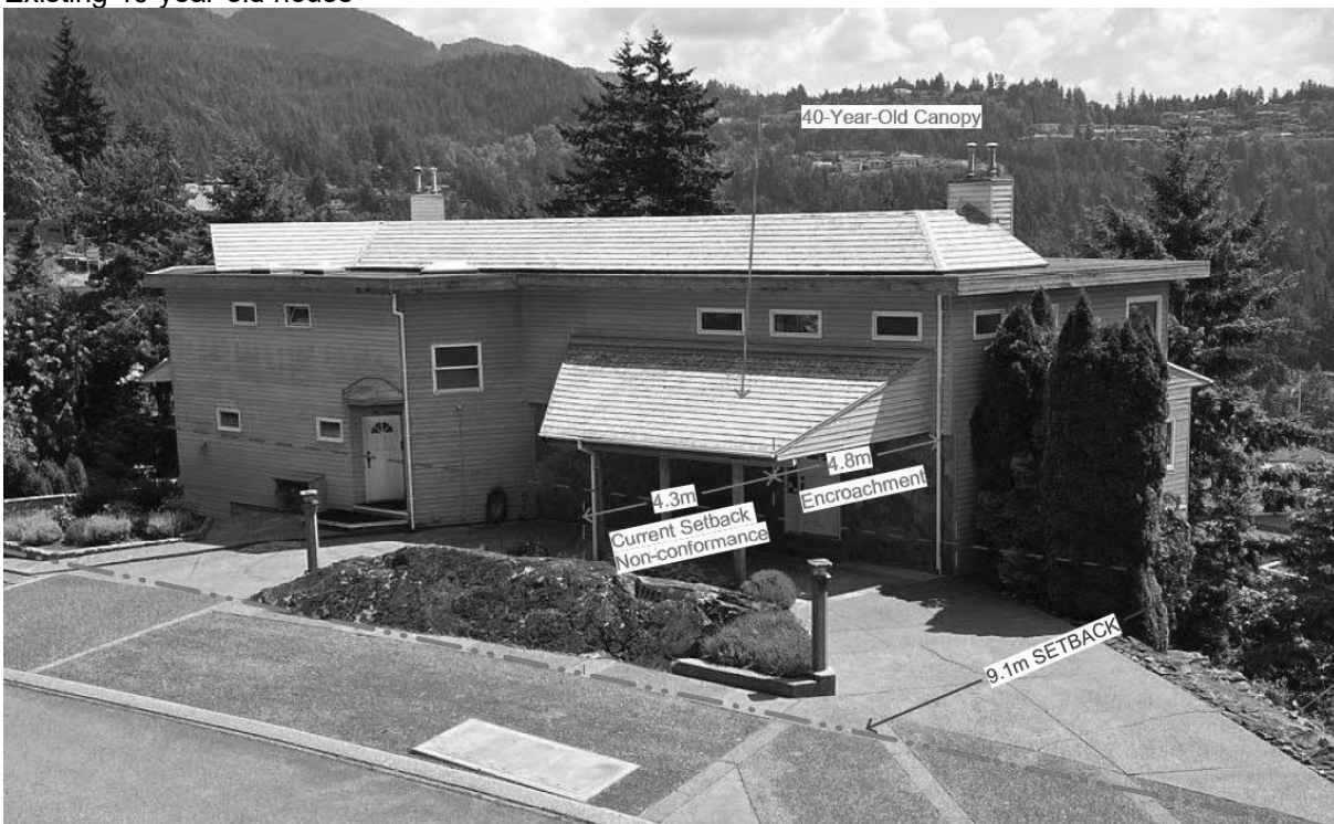
Existing 40-year-old house
