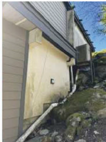
Photo 3: Addition Founded on Bedrock
