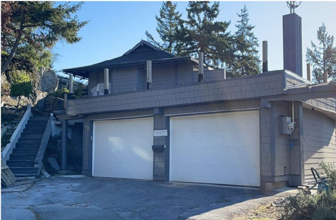
Now (Garage extension has been constructed)
