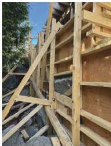
Photo 2: Concrete with Framework
