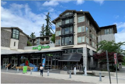
Wesbrook Village, Vancouver
