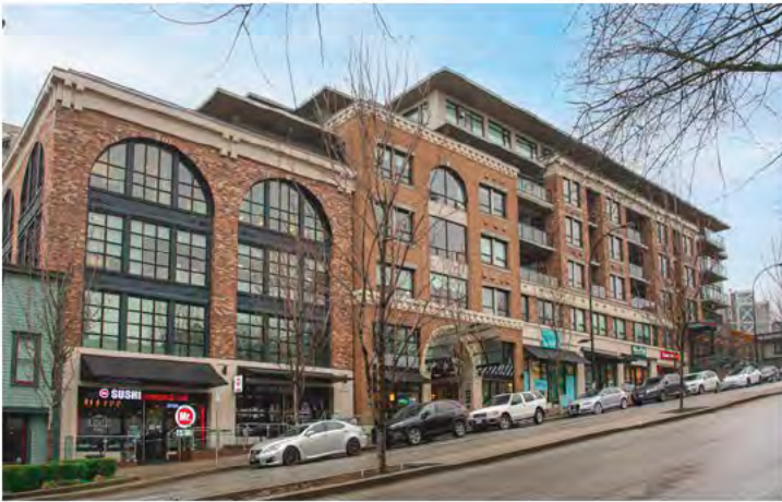
Mid-rise mixed-use can be oriented north-south to better connect the public realm with the waterfront and step building heights with the slope (Lower Lonsdale) | Source: District of West Vancouver
