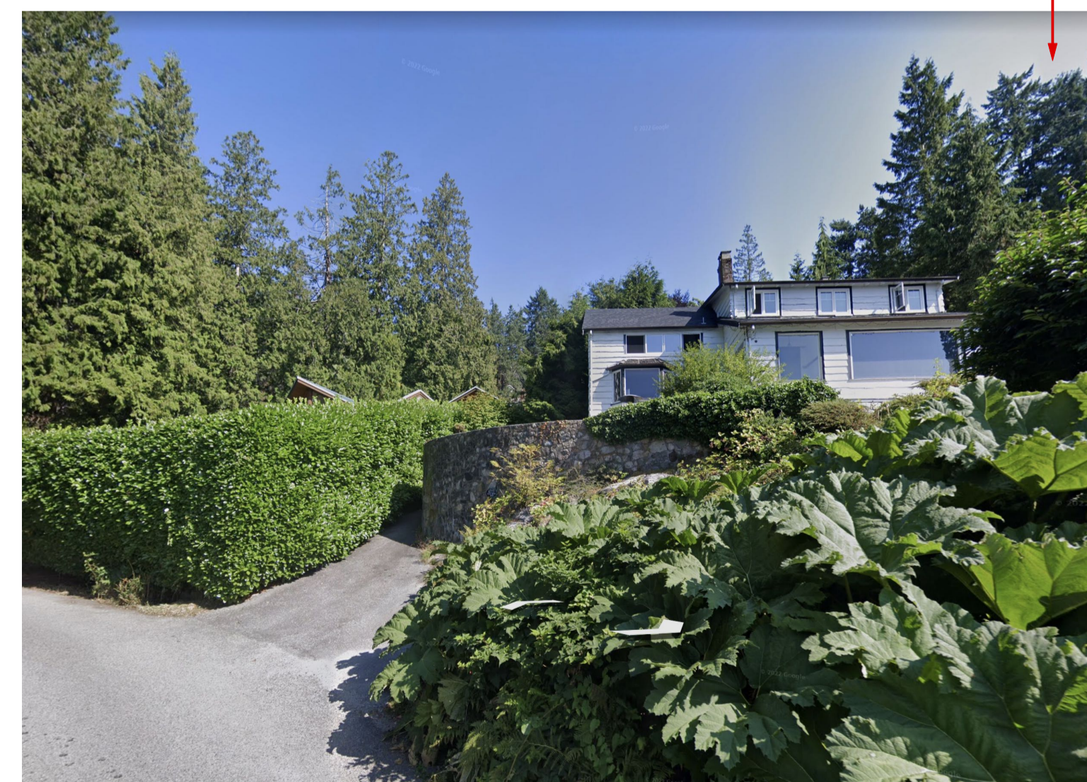
4777 ENTRANCE FROM PILOT HOUSE ROAD
