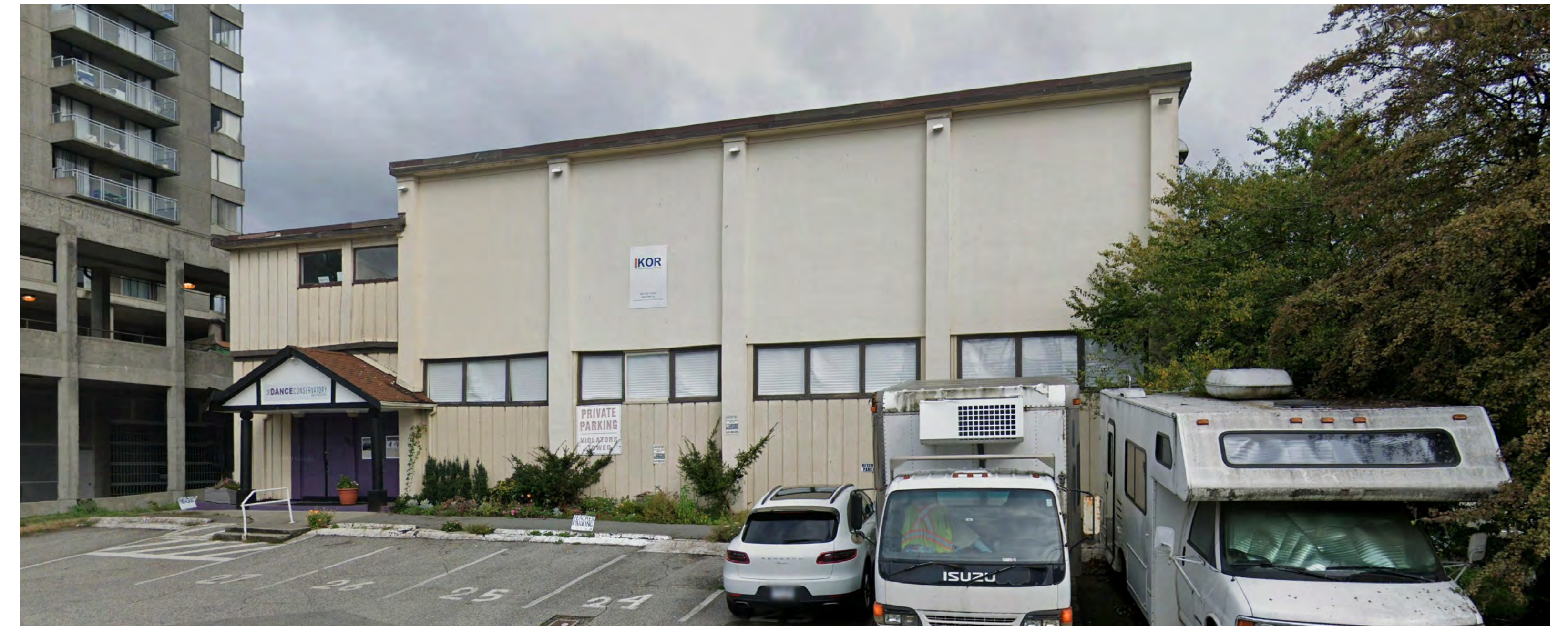
2- STREET VIEW: LOOKING NORTH-EAST
