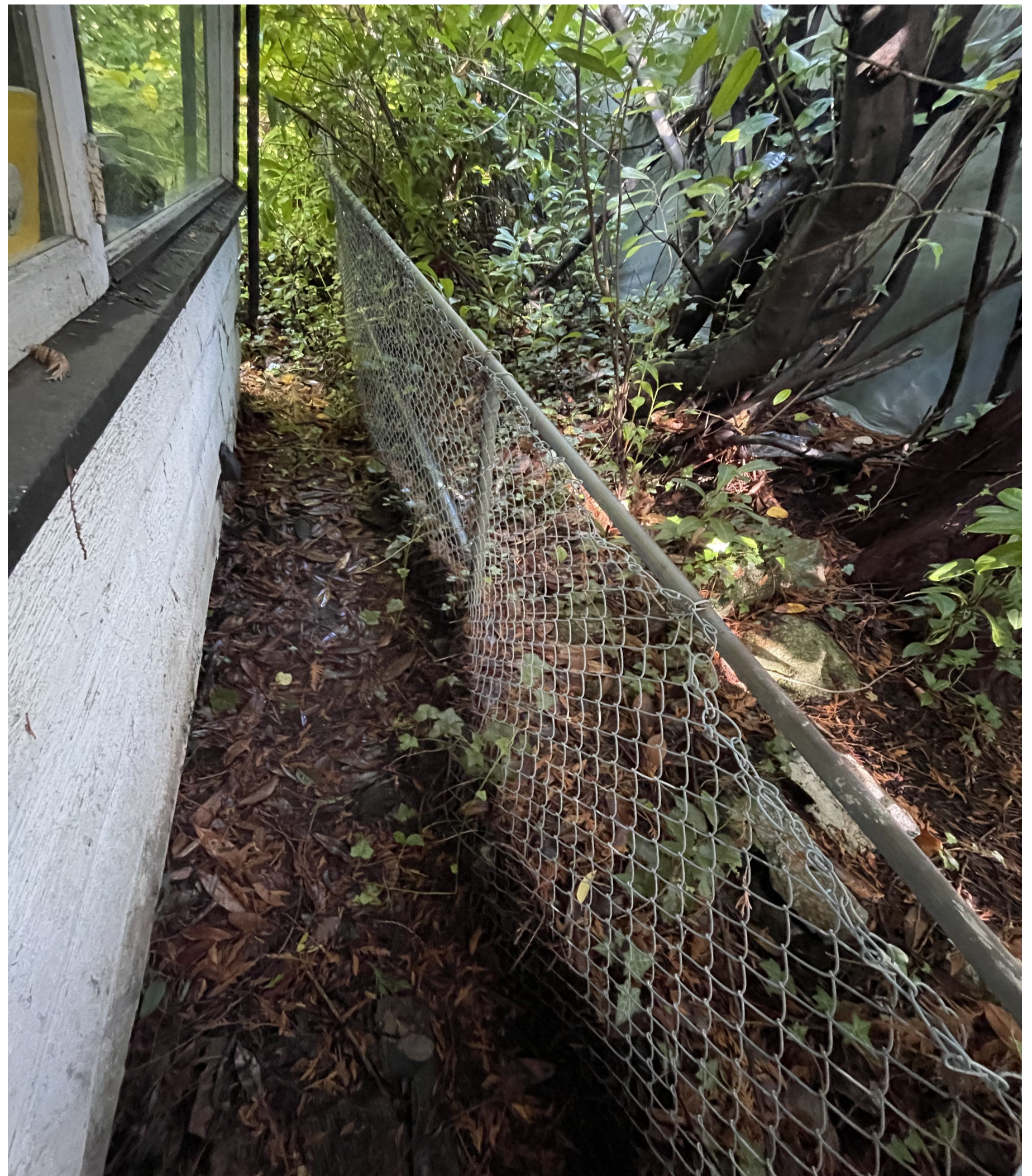
A EXISTING CHAIN LINK FENCE @ 4777 PILOT HOUSE Rd EAST PROPERTY LINE BETWEEN 4777 & 4775
