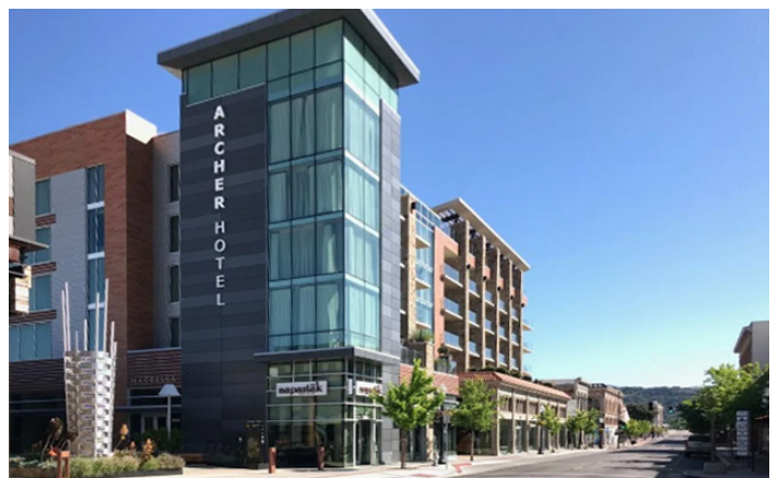
Specific uses with distinctive architecture, such as a mid-rise hotel, can become focal points and landmarks for both visitors and locals (Napa) | Source: Napa Valley Register
